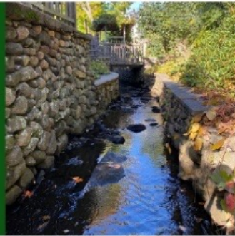
retaining wall condition
