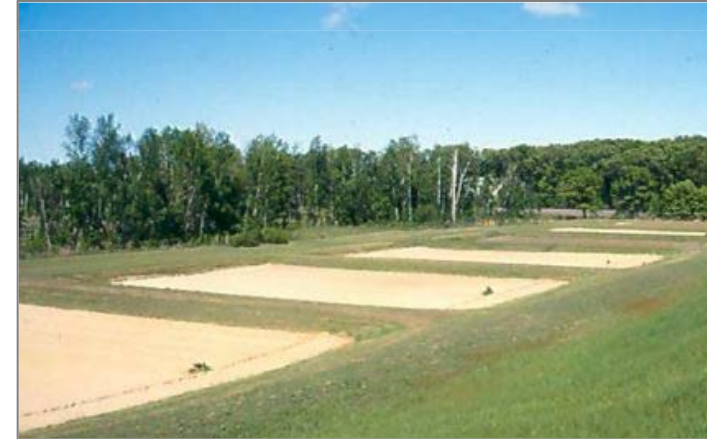
Rapid Infiltration Basins
