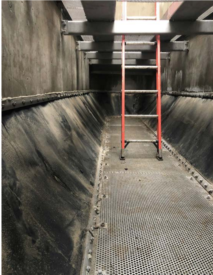
View looking down filter cell at top perforated plate
