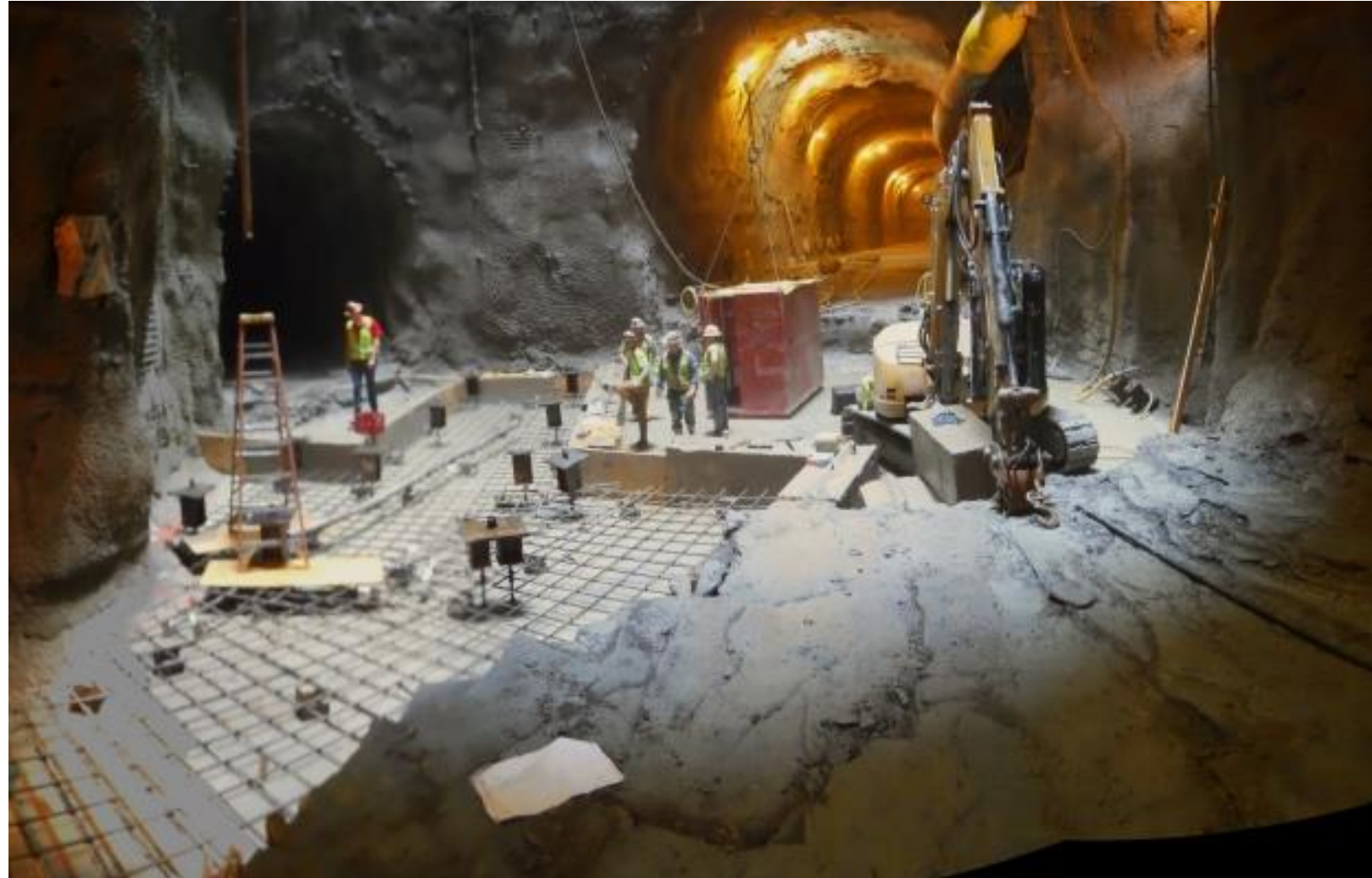
Euclid Creek Tunnel, Cleveland, OH
