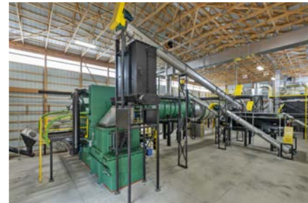
Morrisville, PA (2019) • 35 wet ton/d • Fluid Lift Reactor
