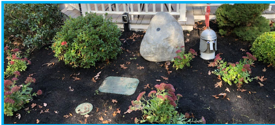
Landscaped Air Pump and Controls
