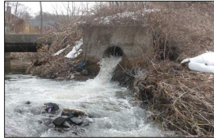
Structural Overflow to River
