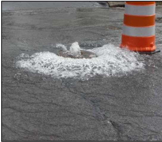
Overflow from Manhole
