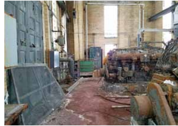
Pump station pre-restoration
