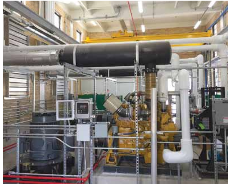
Lowell's restored flood pump station
