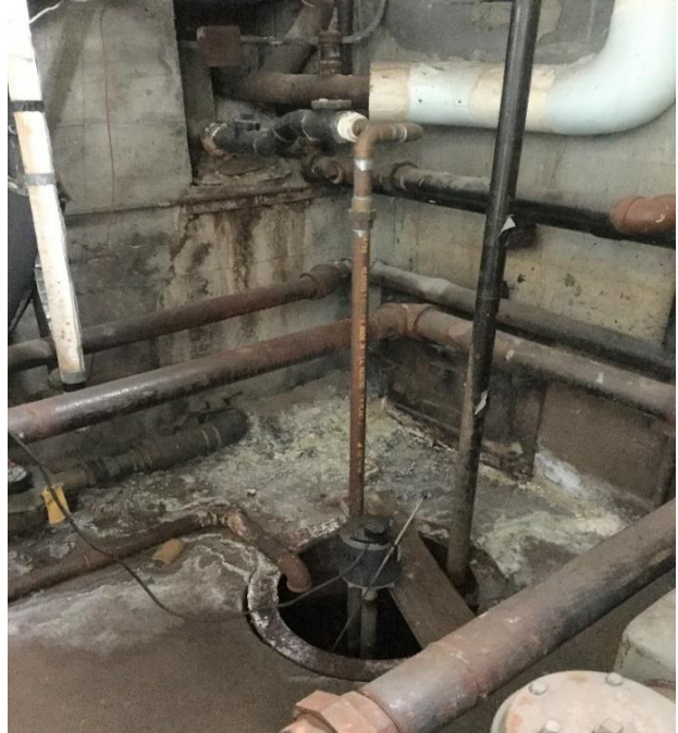
Photo 3 - Sample of Illicit Connection (Sump Pump to Sewer - Image by Weston & Sampson)
