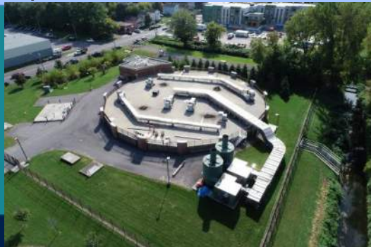
Lower Harbor Brook Storage Facility
