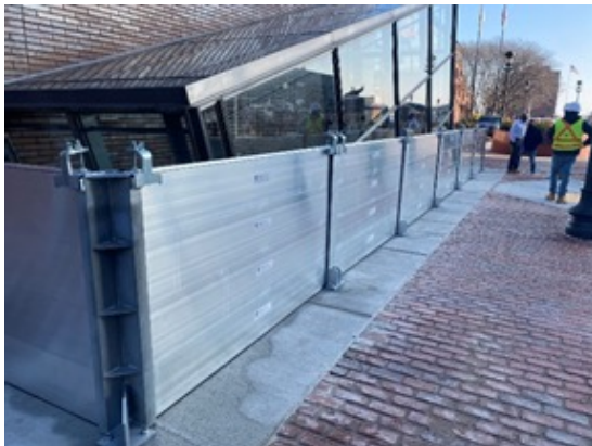
Stop Logs, Aquarium Station, Boston, MA
