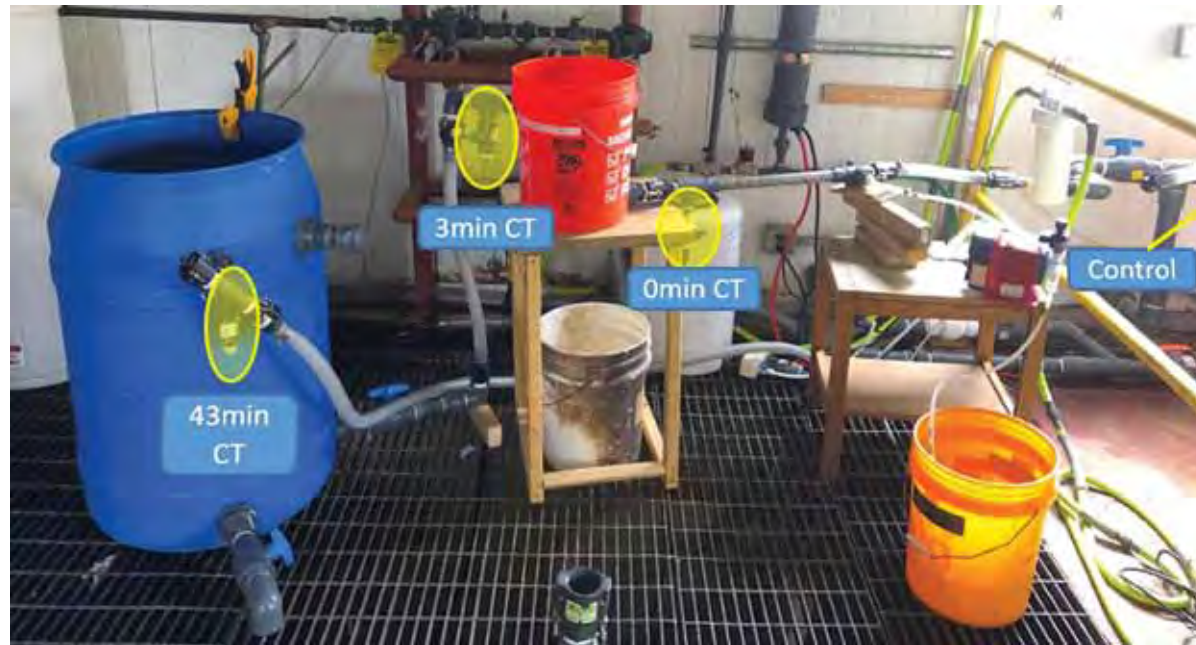
Figure 4. Pilot flow-through disinfection setup
