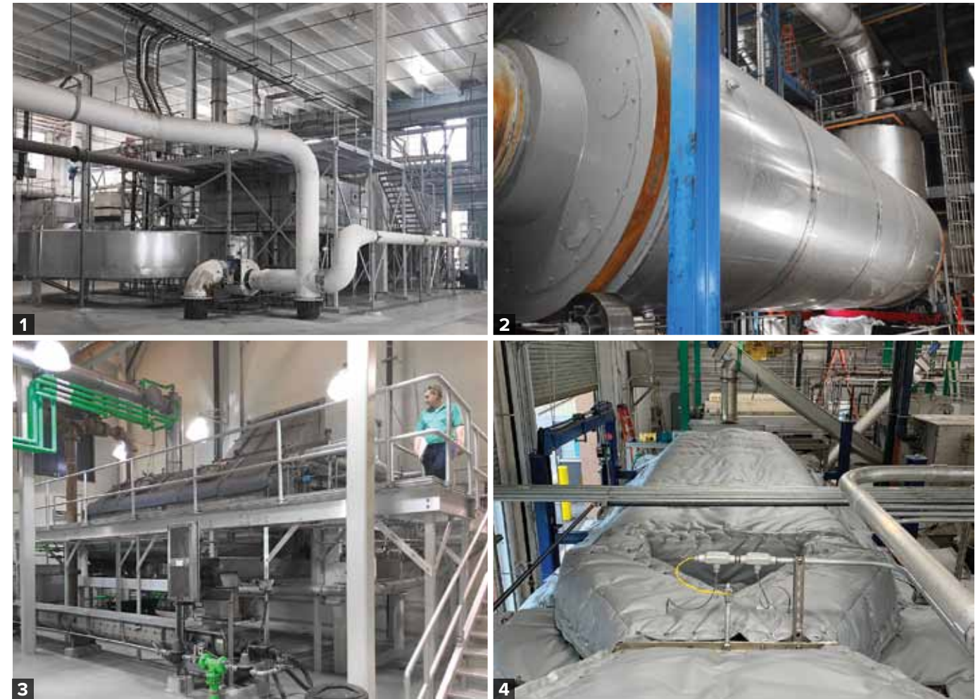
1. Belt dryer installed at the Western Wake Regional Water Reclamation Facility in New Hill, NC 2. Drum dryer installed at the Massachusetts Water Resources Authority Residuals Pellet Plant in Quincy, MA 3. Paddle dryer installed at the Derry Township Municipal Authority Clearwater Road Wastewater Treatment Facility in Hershey, PA 4. Belt dryer installed at the Chalfont-New Britain Township Joint Sewage Authority's Advanced Wastewater Treatment Facility in Doylestown, PA
