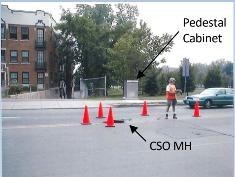
N-22 Pedestal Cabinet and Overflow Manhole
