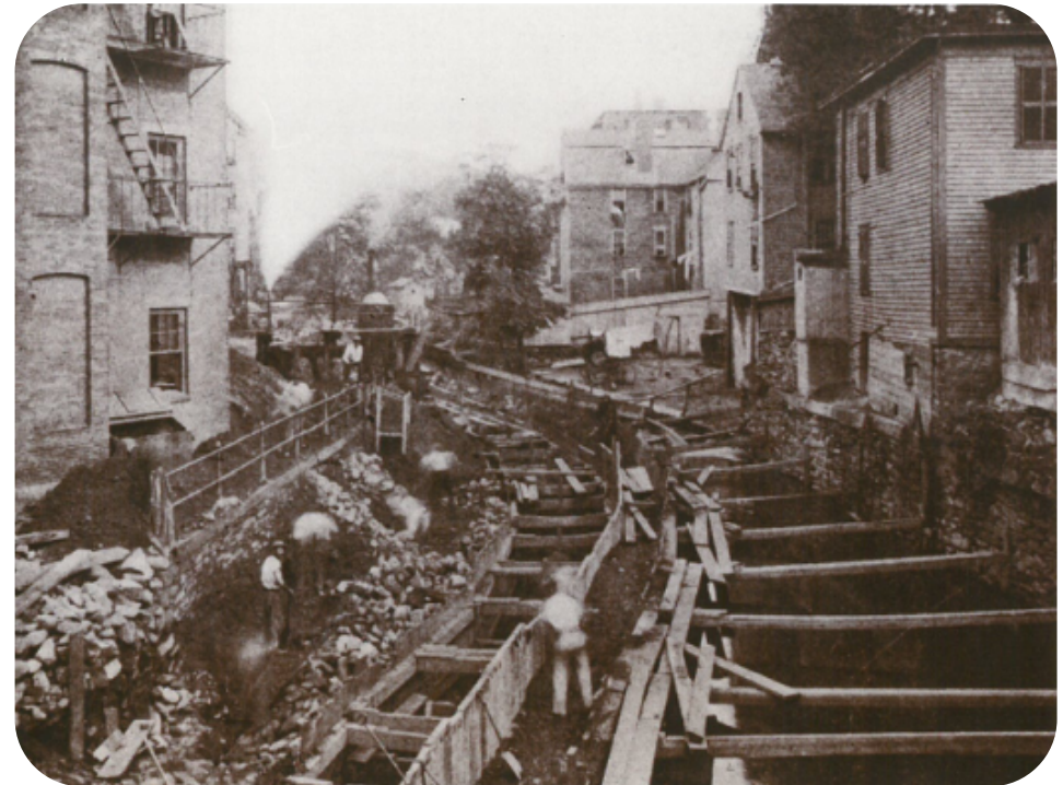
Moshassuck River Interceptor Construction circa 1897
