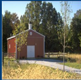
Small Community On-site Wastewater Treatment 40 homes; Agriculture/ Open Space Preservation.
