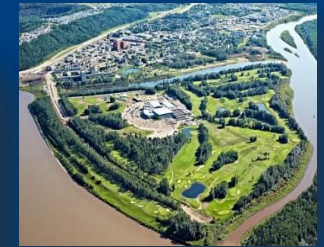
MacDonald Island, AB, Canada Integrated Water Reuse and Heat Recovery system utilizing treated wastewater effluent for irrigation and flush water while also recovering the effluent heat for pool heating within the rec center.
