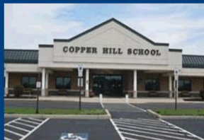
Copper Hill Elementary School, East Amwell, NJ 1 st public school water reuse system
