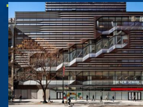
The New School University, NYC 40,000 GPD in-building onsite water treatment & reuse for flushwater, cooling, irrigation & laundry.
