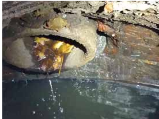
Gray filamentous algae in seepage at a pipe penetration in a stormwater catch basin often indicate indirect illicit connections
