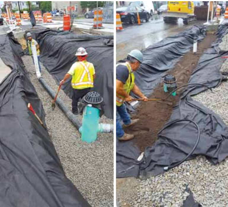
Bioretention basin—installation of crushed stone layer with perforated underdrain, cleanout, and overflow structure, (right) bioretention soil storm sewer main. An approximately 2,830 ft (863 m) of 6.5 ft (2.0 m) wide porous asphalt cycle track and 9,000 ft 2 (837 m 2 ) of permeable concrete unit pavers will be installed.
