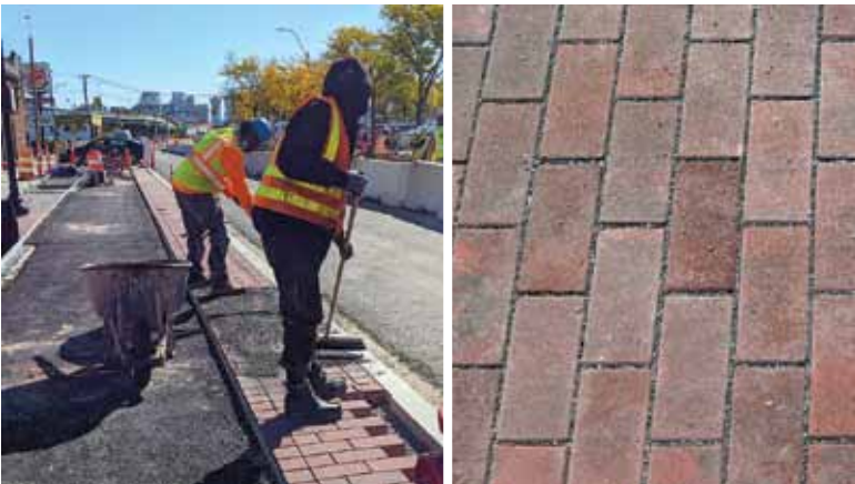
Paver installation crew sweeping the joint filler stone into the spaces between the pavers. Infiltration testing performed after sweeping the joints verified that the installation met the specified infiltration rate. (right) Closeup showing the 1/4 in. (0.64 cm) stone used for joint filler.
