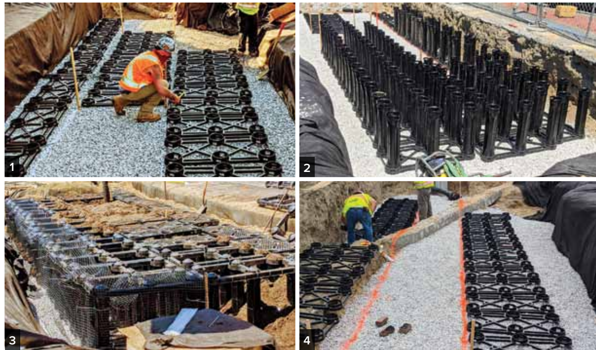
Soil Cell installation: (1) Worker carefully spaces the bases on the aggregate subbase. Once the spacing is verified, the base plates are nailed into place. (2) Posts have been installed, six posts to each base plate. (3) Strongbacks installed to restrain the posts while planting soil is placed within the cell and stone is placed outside the cell. (4) Strongbacks replaced by decks. Crushed stone placed over the planting material.
