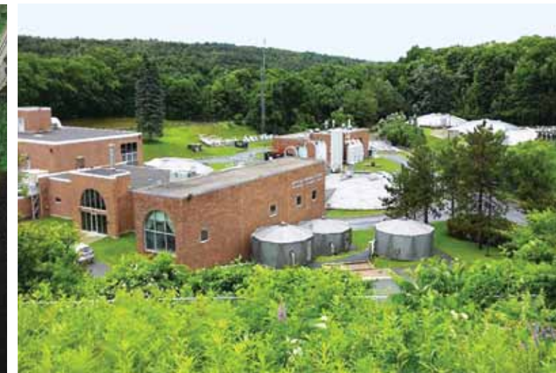
The Greater Augusta Utility District's wastewater treatment plant
