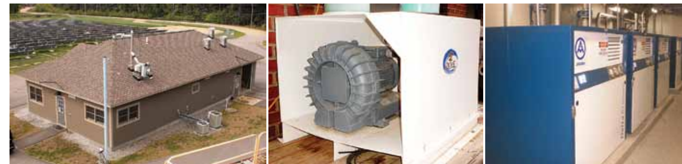
Pheasant Road influent pump station
