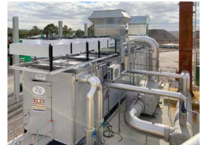
Exterior of CHP engine installation
