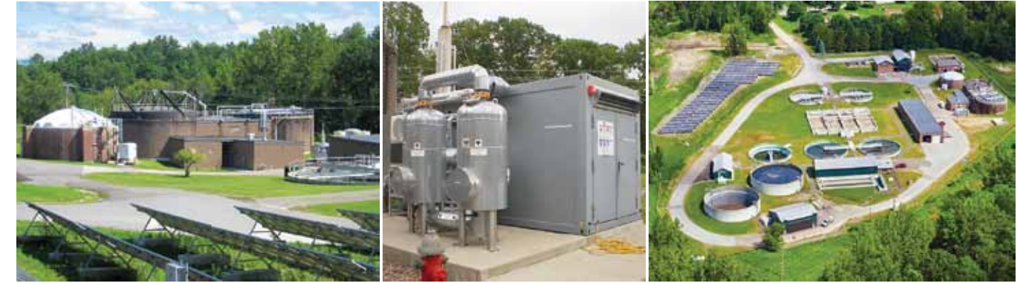
Anaerobic digester complex with solar panels in foreground
