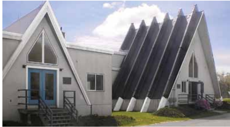
Plymouth Village Water and Sewer District facility
