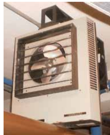
Headworks electric unit heaters
