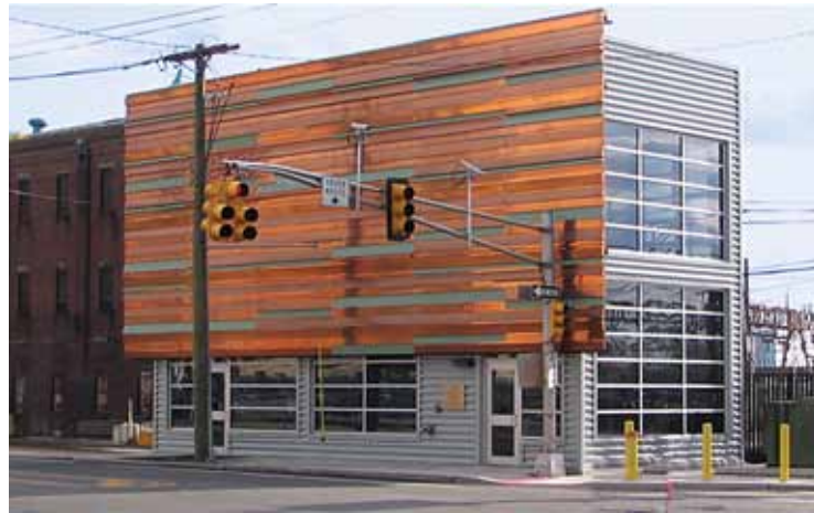
Photo 1. H1 wet weather pump station
