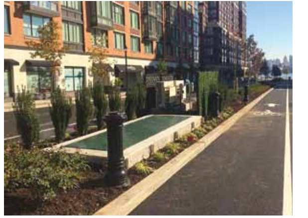
Photo 3. H5 wet weather pump station electrical vault
