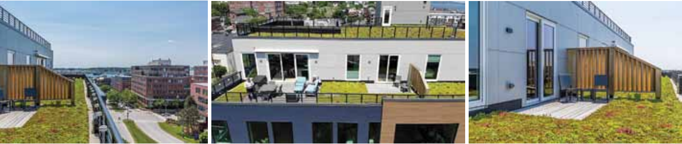
The Luminato condominium project is the first green roof constructed within the zone
