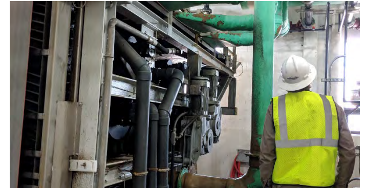
2-M belt filter press at Gresham WWTP
