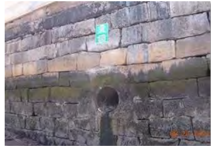
Closed outfall (top), former CSO discharge that now discharges stormwater, only (bottom)
