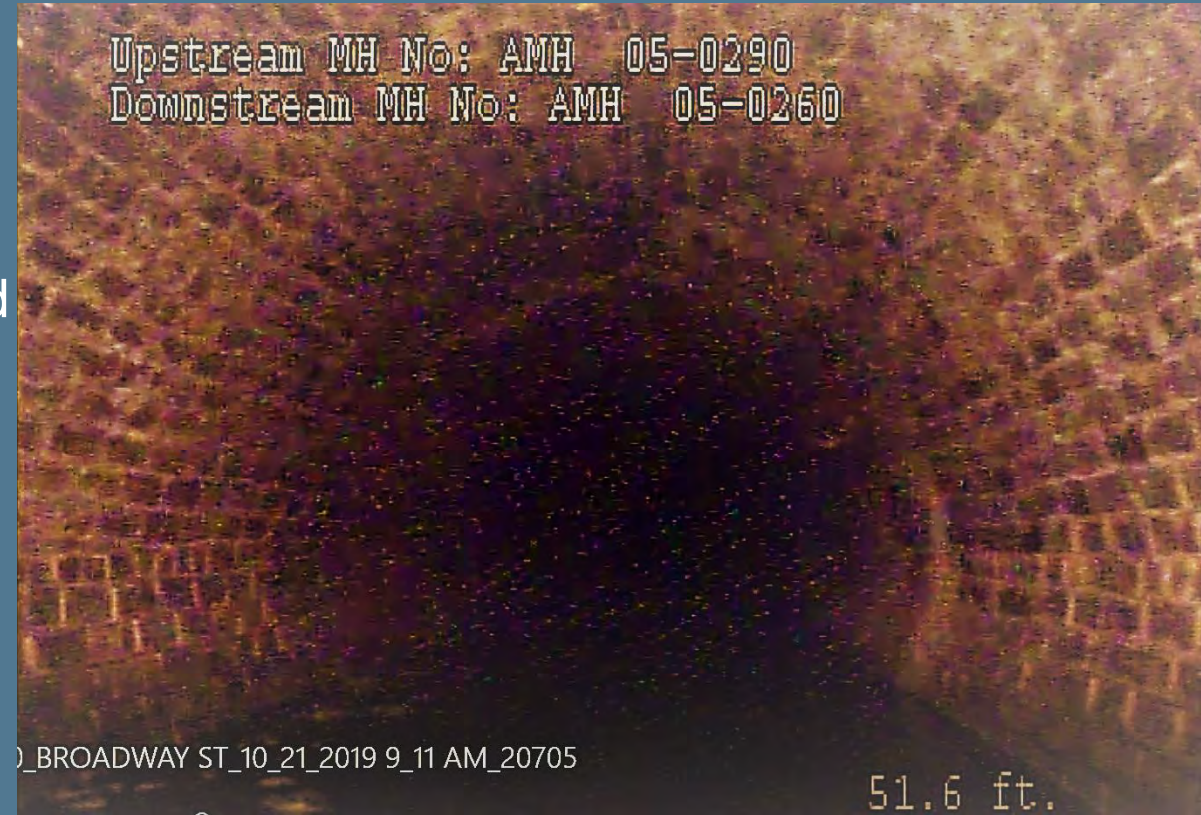
72-inch combined sewer along Broadway
