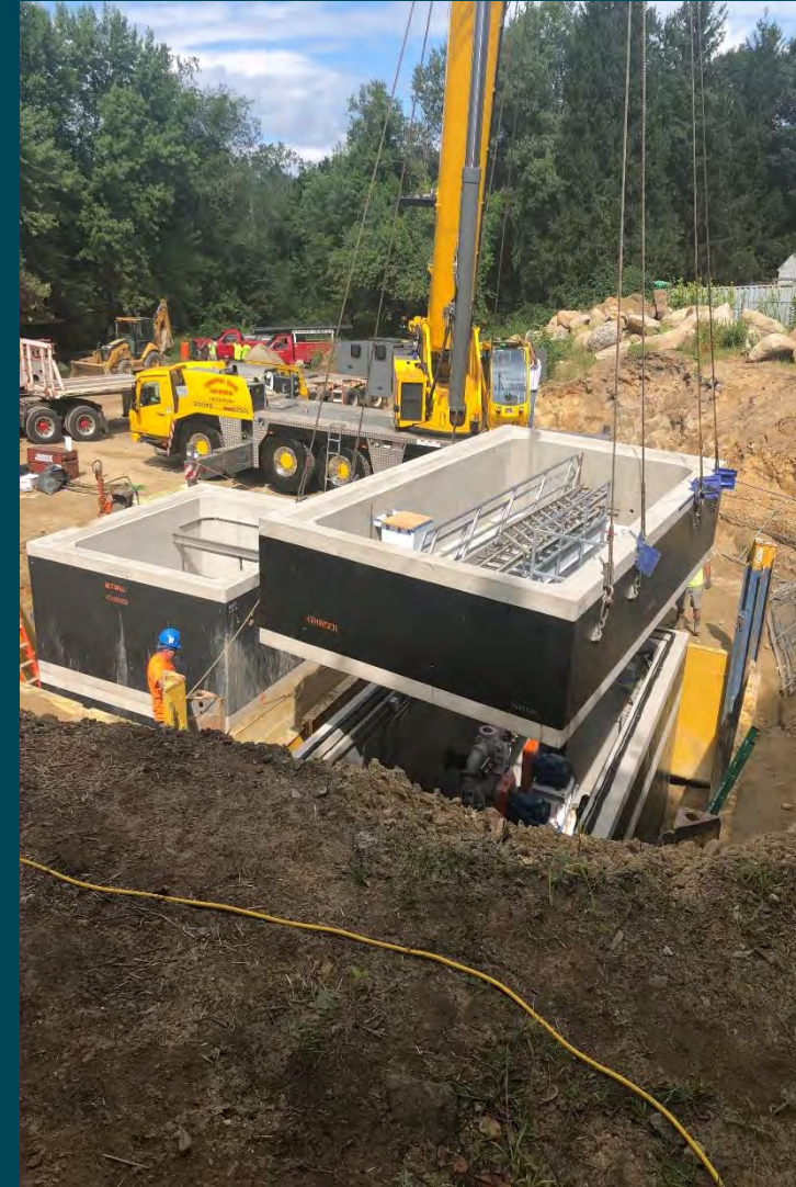
Install of Pump Station Sections
