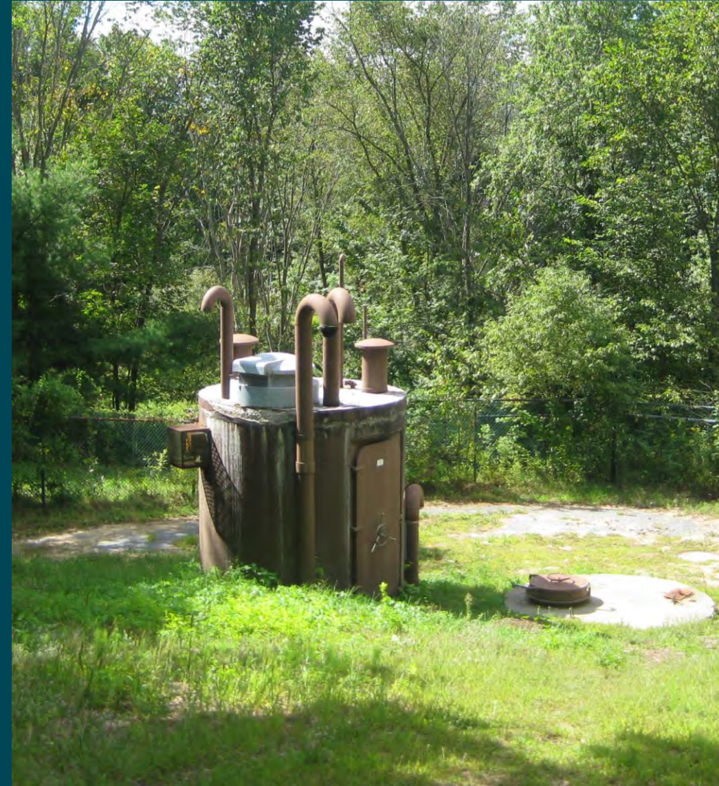
Existing pump station in flood plain on federal lands
