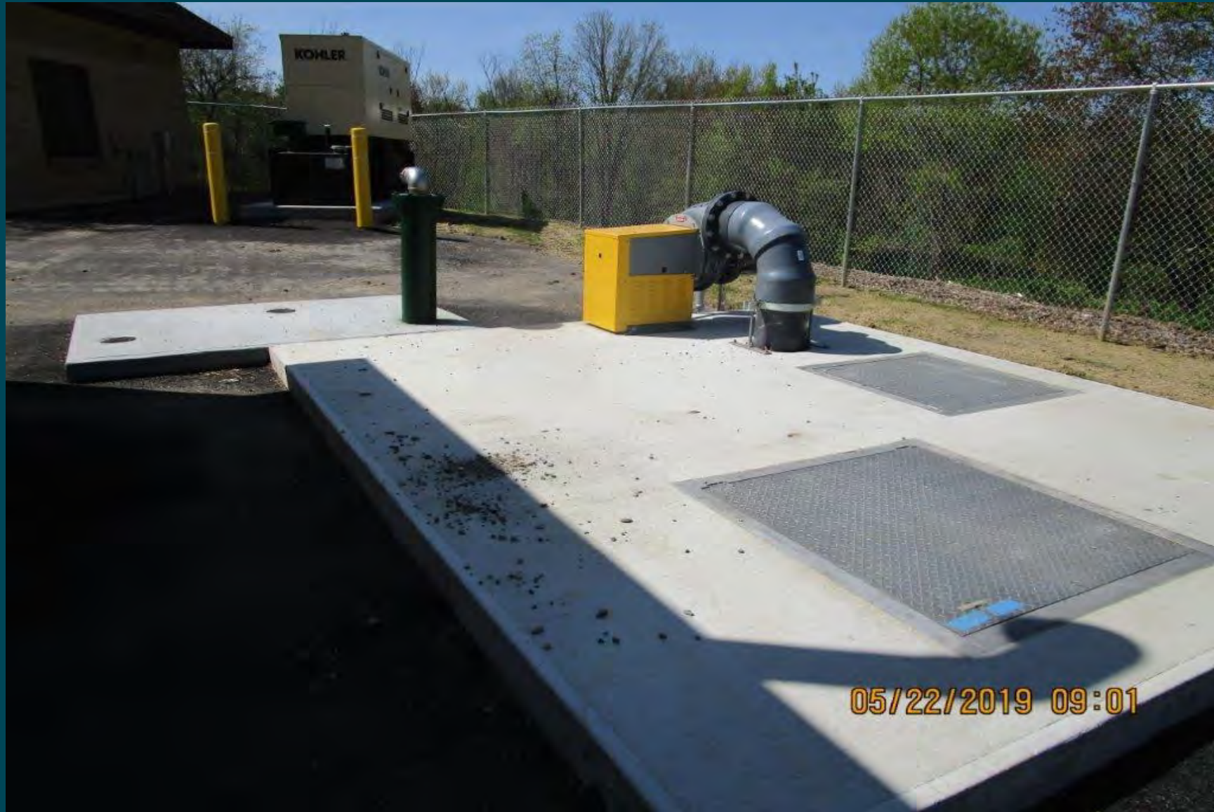
Wet Well Top Slab
