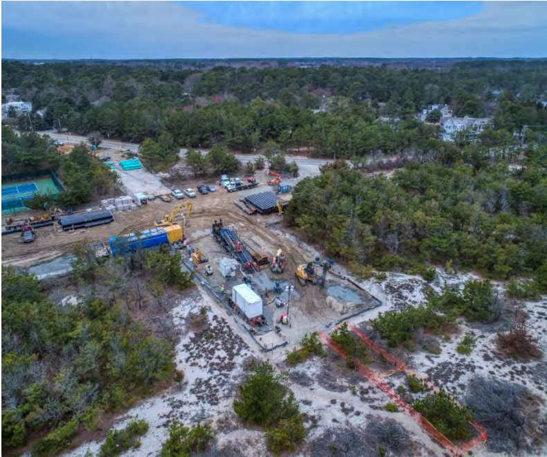
Horizontal Drilling at Deauville Beach
