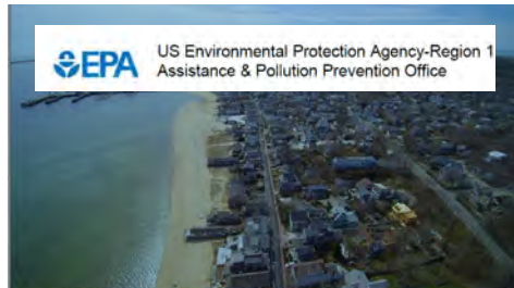
Provincetown Stormwater Program Revitalizes Downtown and Improves Beach Water Quality using Porous Asphalt
