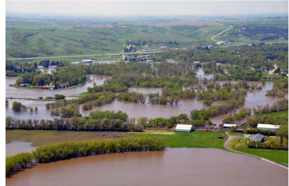
Flooding in Souris River Basin June 2011. USACE Photo
