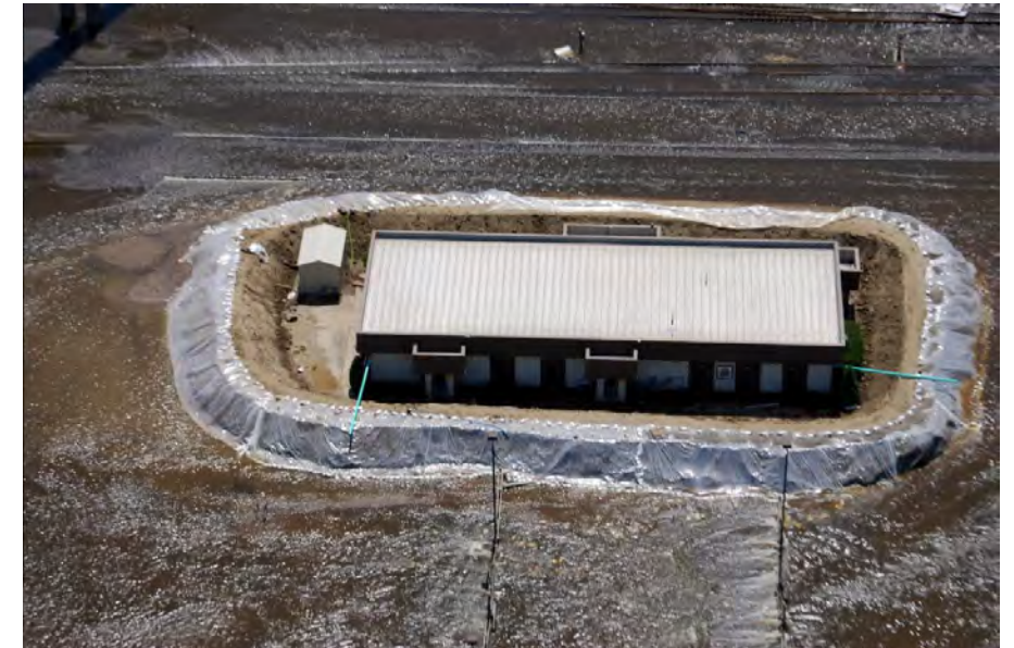
June 2011 damages reduced by City of Minot, USACE, USFWS, and National Guard. USACE Photo
