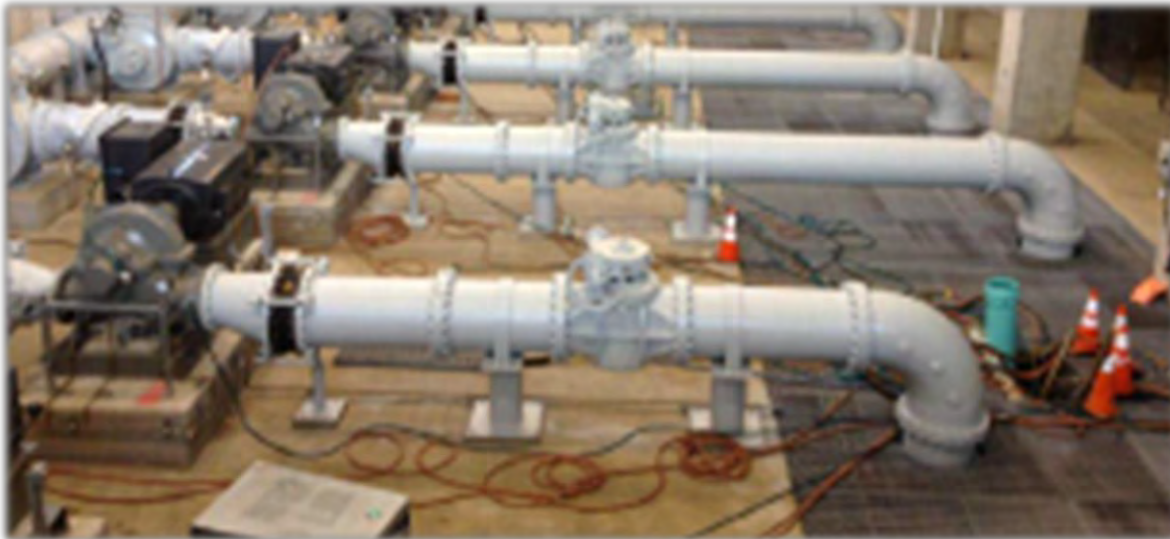
Existing Suction Piping with Eccentric Reducer at Pump Suction Nozzle
