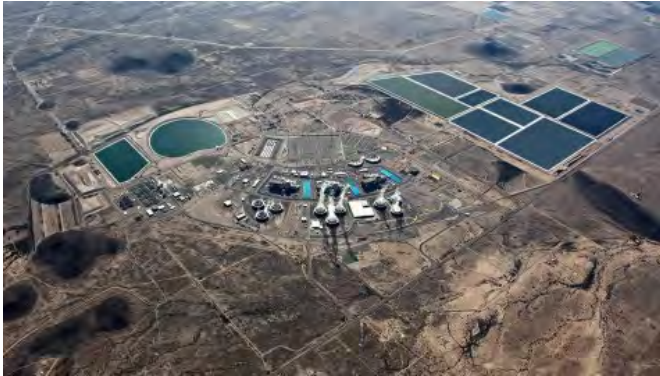
Palo Verde Power Station Arizona
