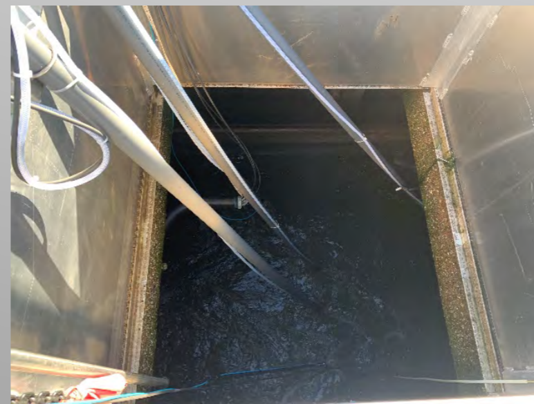
View into tank
