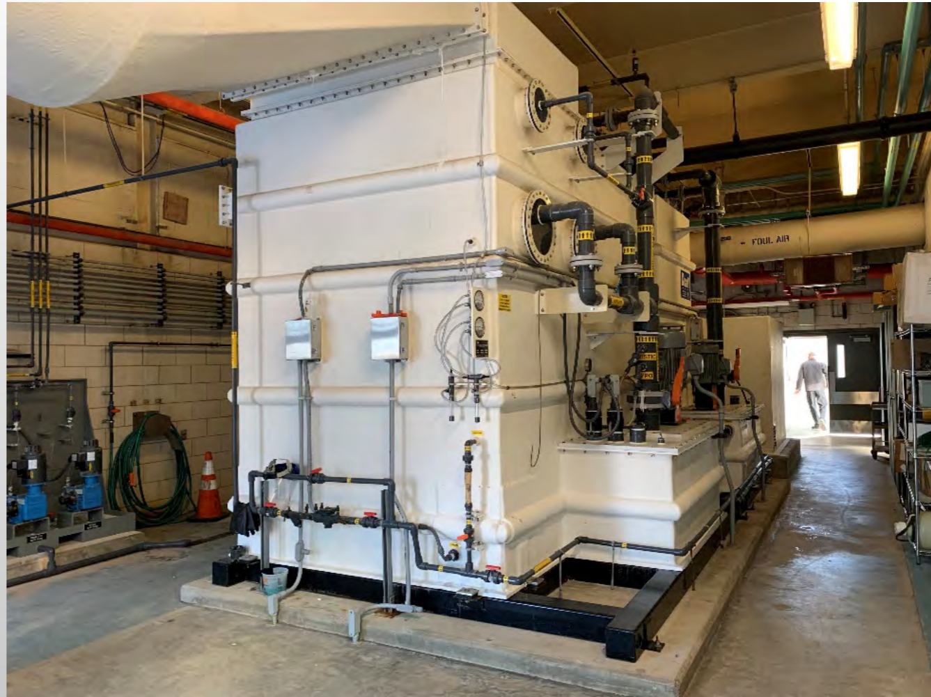
Odor control room
