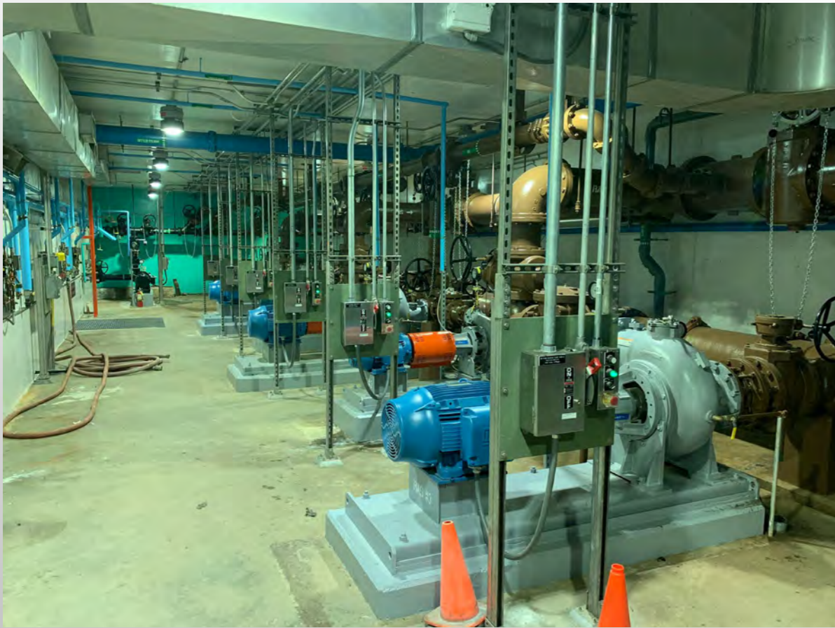
Secondary sludge pumps and piping
