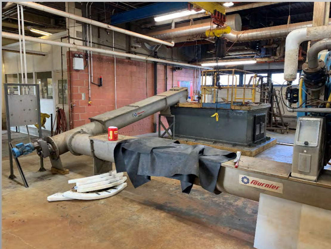
Auger from Fournier presses to hopper
