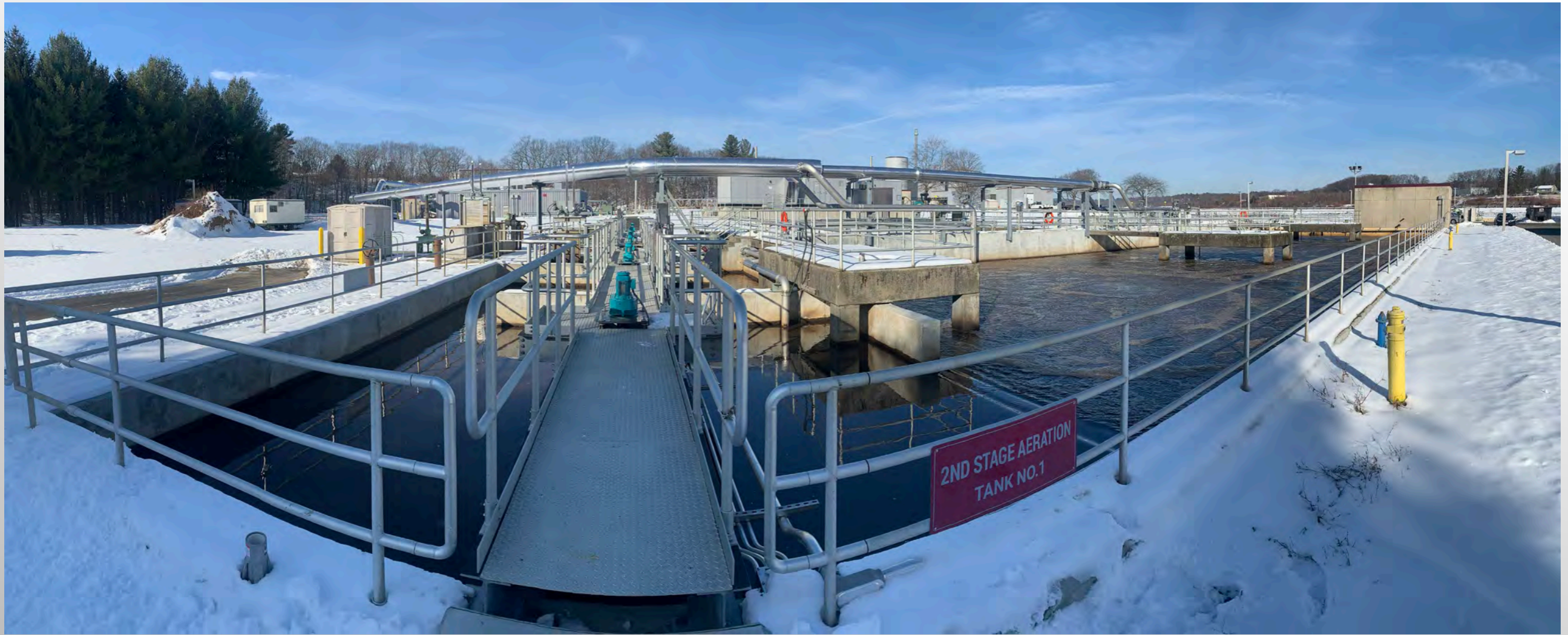
Secondary treatment, 2nd stage aeration tanks
