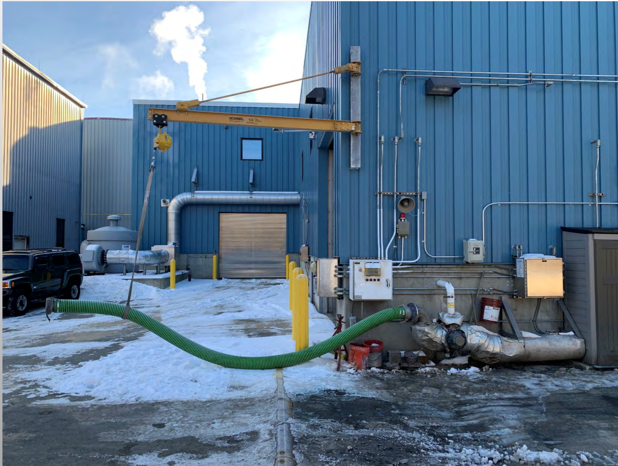
Septage disposal station
