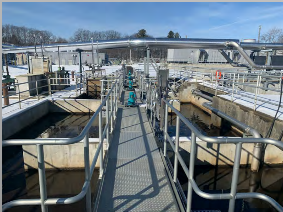
Secondary treatment, 2nd stage aeration tanks
