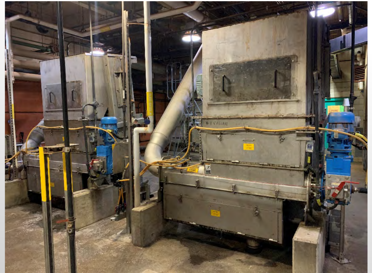
Mechanical bar screens, screenings washer, and compactor presses
