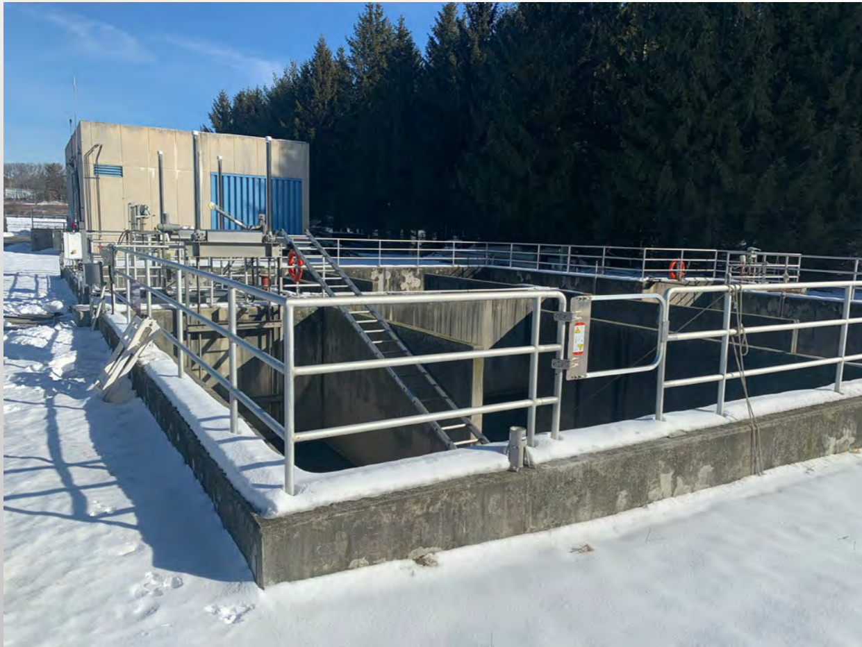
Chlorine contact tanks and chlorine building
