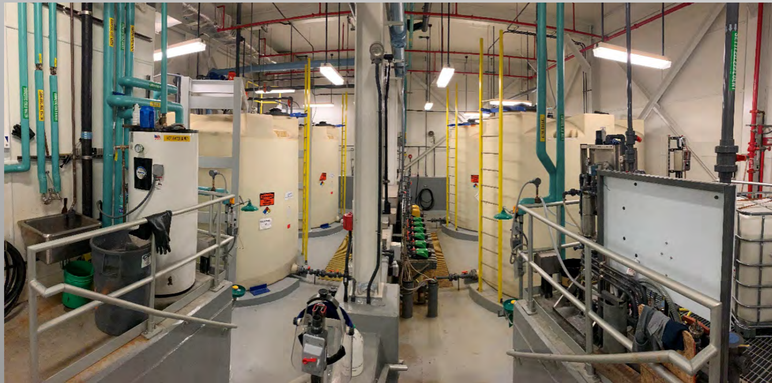
Chemical Enhanced Primary Treatment (CEPT) Room
