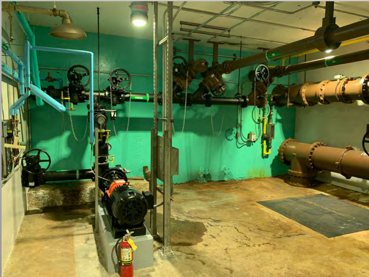
Secondary sludge pumps and piping
