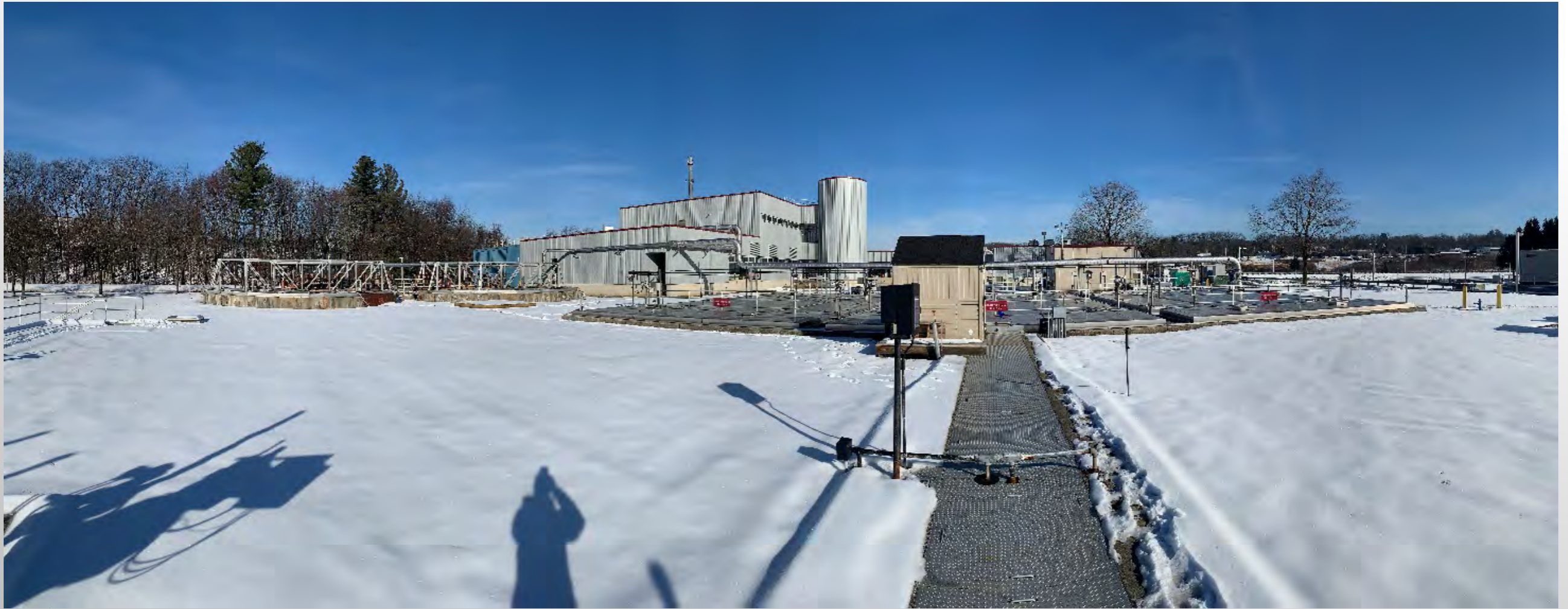
Primary settling tanks (#1-3)
