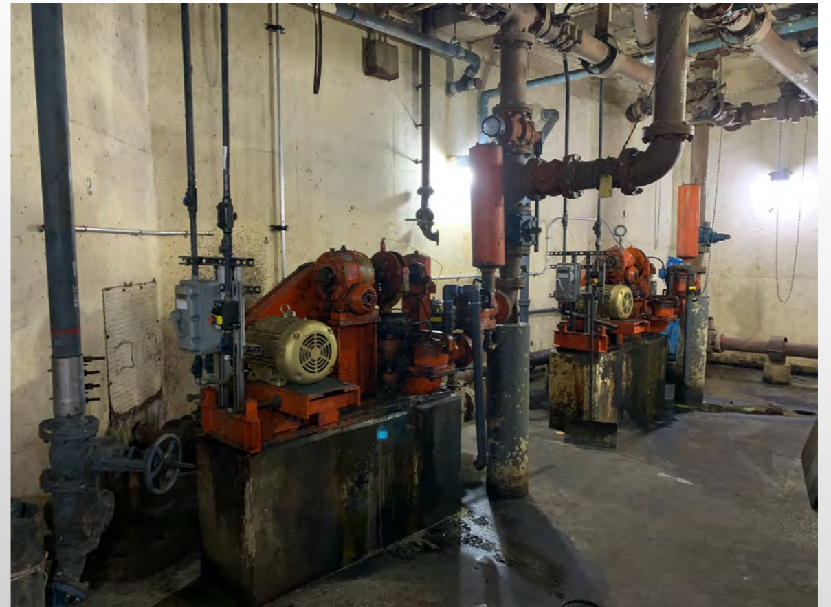
Primary sludge pumps
