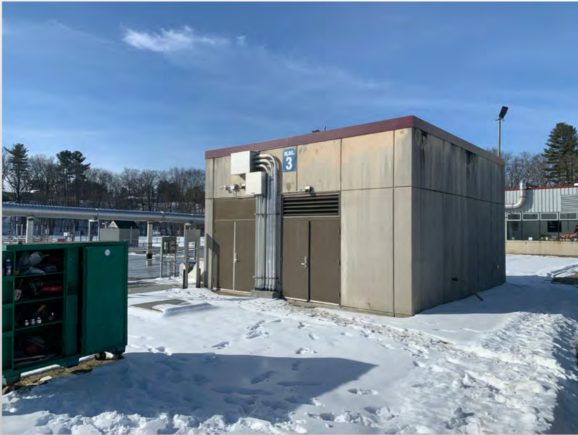
Primary pump gallery access building
