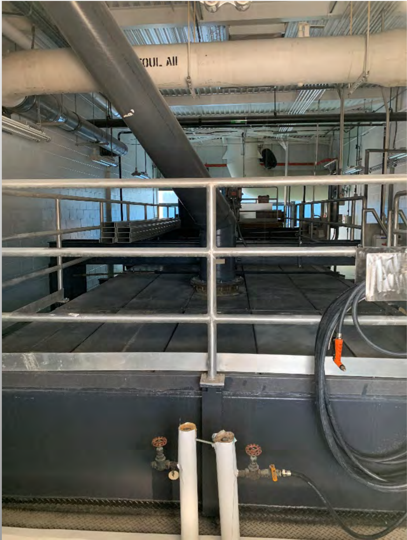
Sludge blend tank
