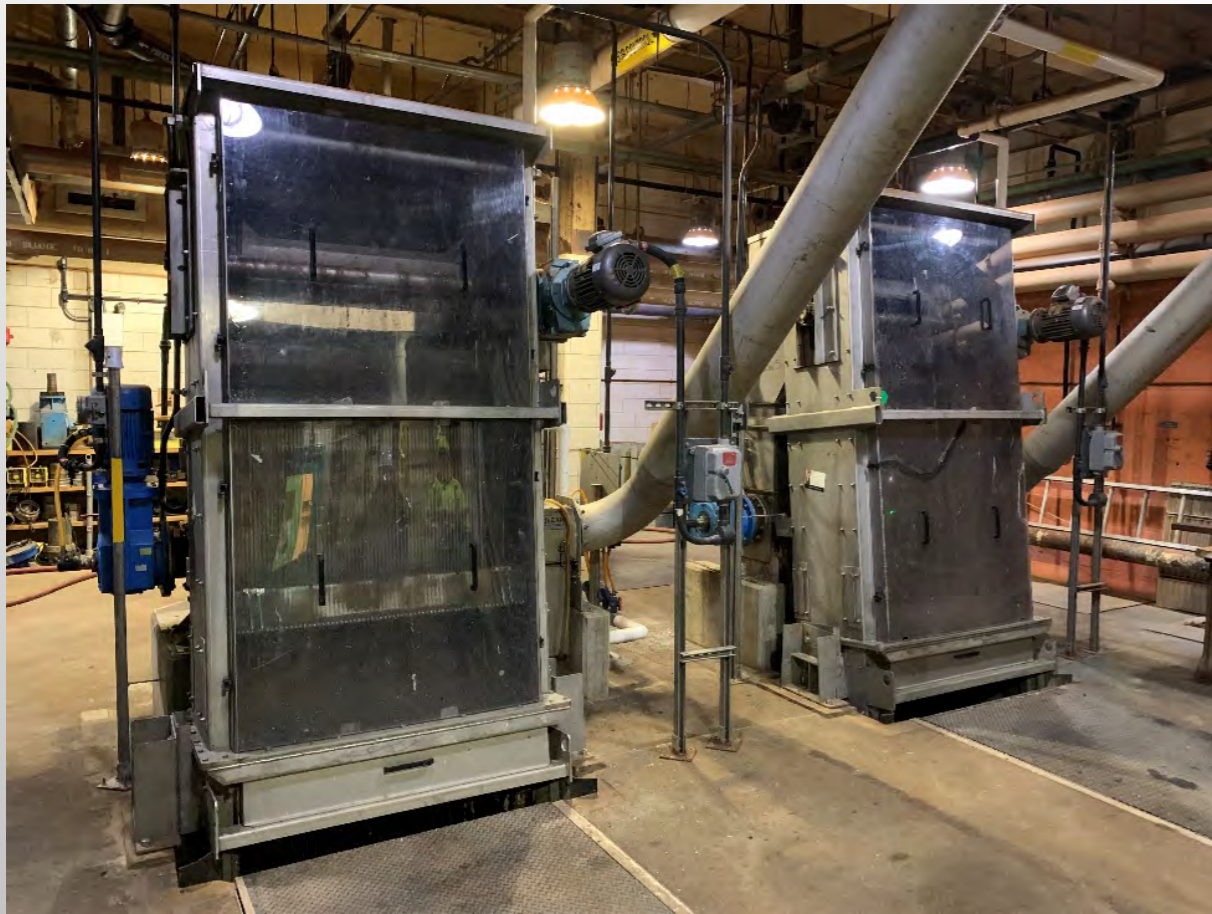
Mechanical bar screens, screenings washer, and compactor presses
