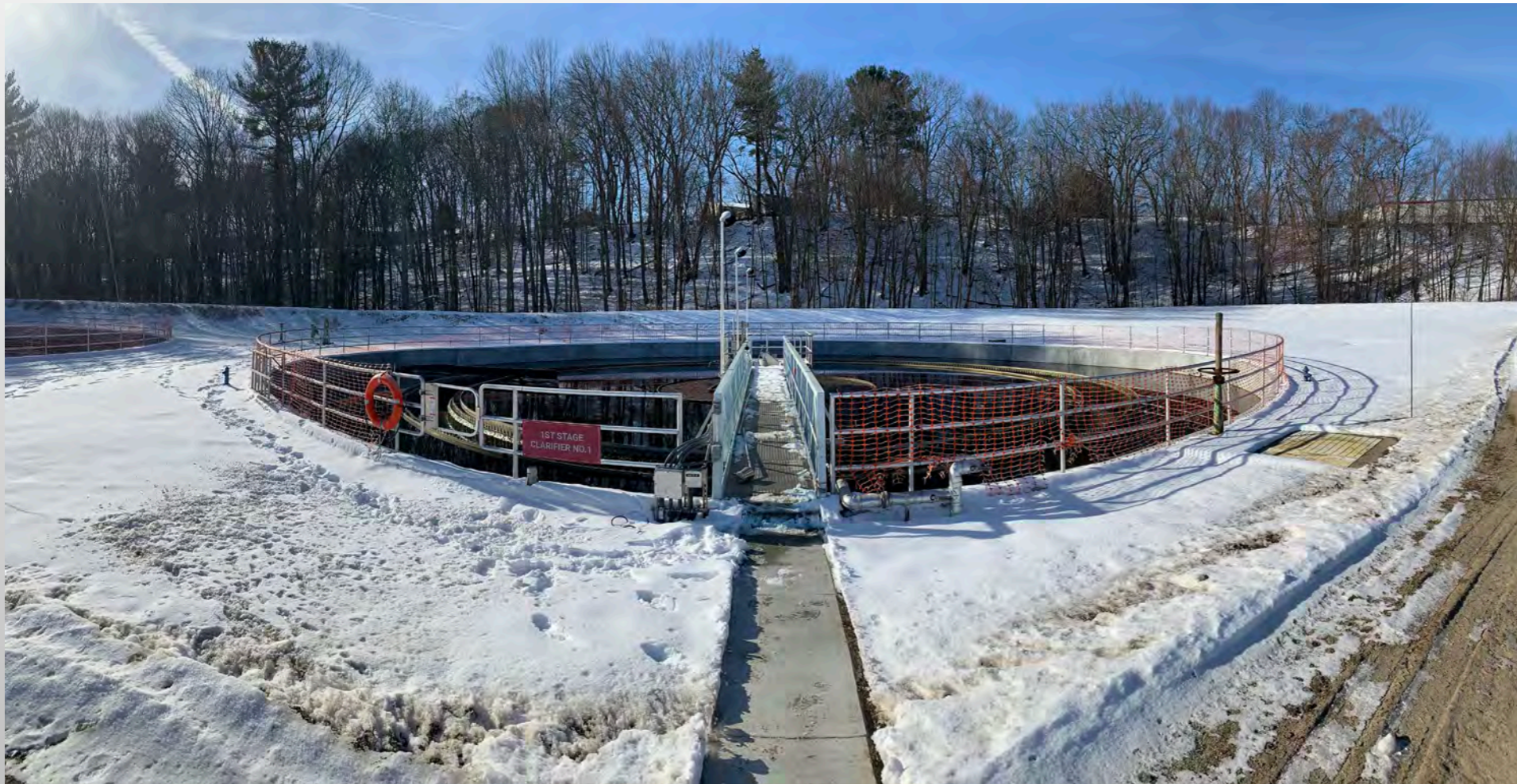
Secondary treatment, 1st stage clarifiers
