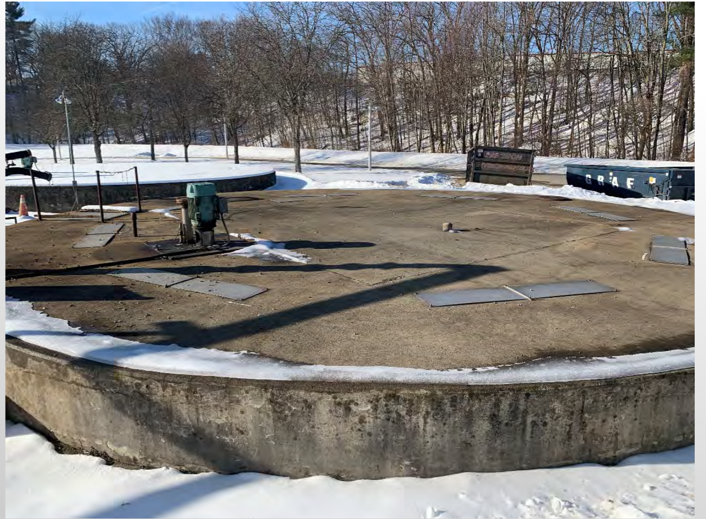
Sludge holding tank (1 of 2)
