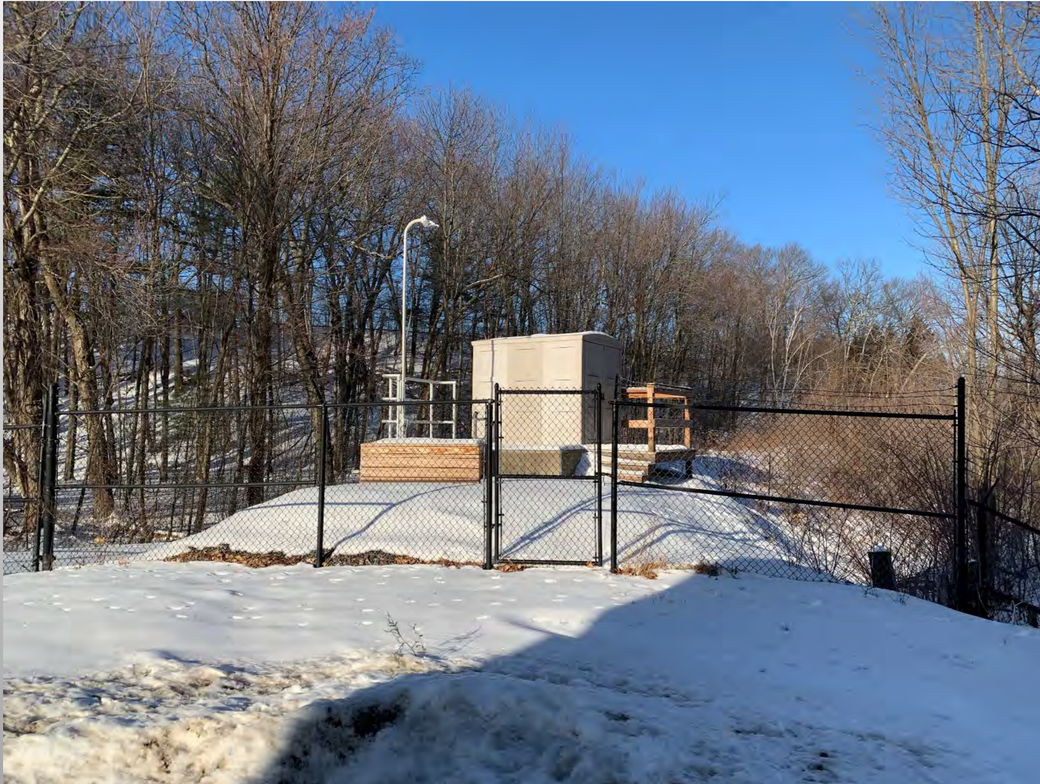
Sampling shed/influent from the collection system
