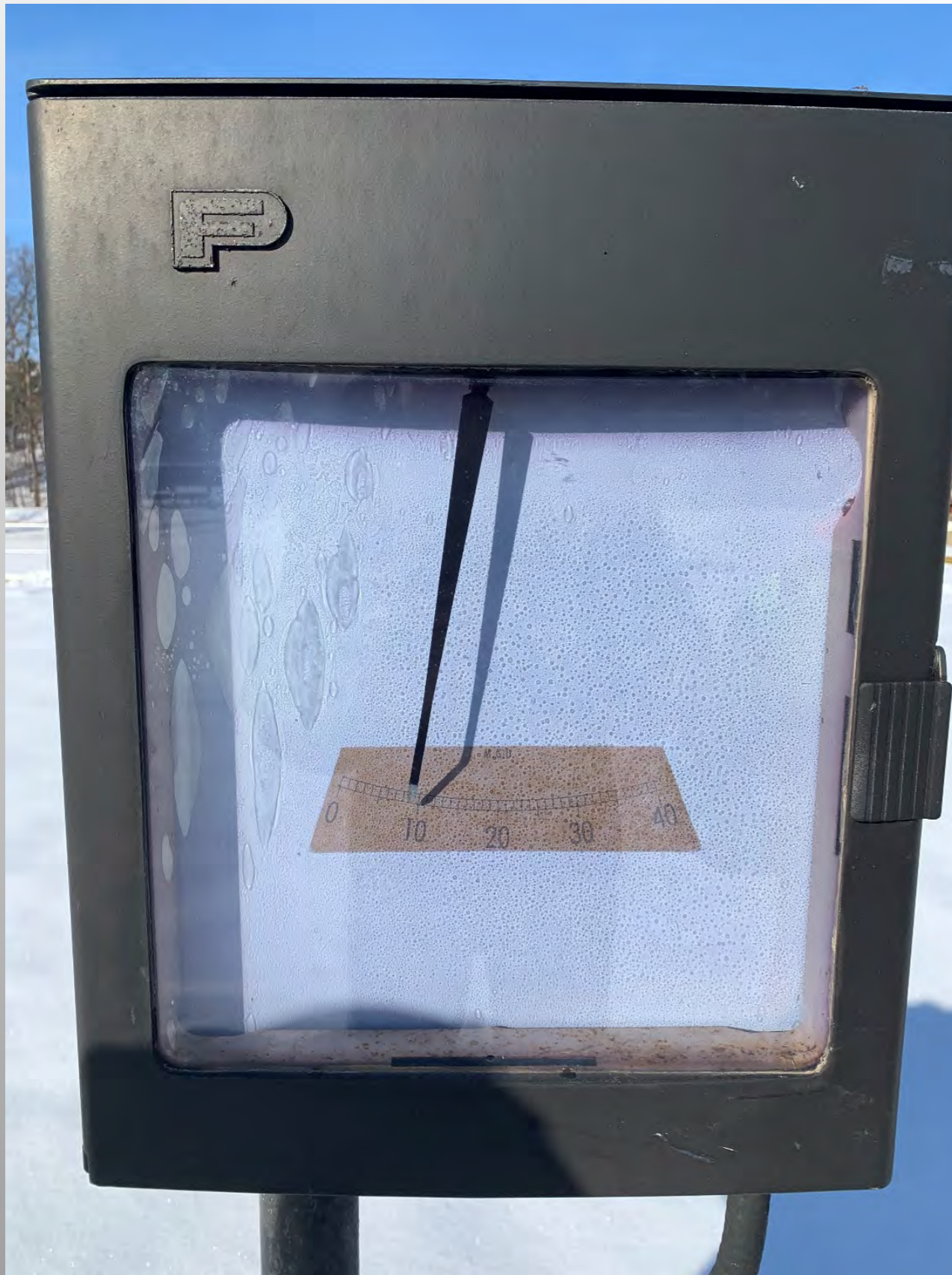
Primary effluent flow meter (note 40 MGD max.)
