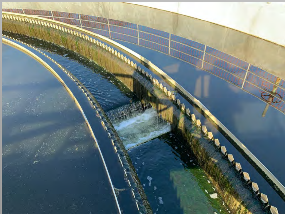
Secondary treatment, 1st stage clarifiers
