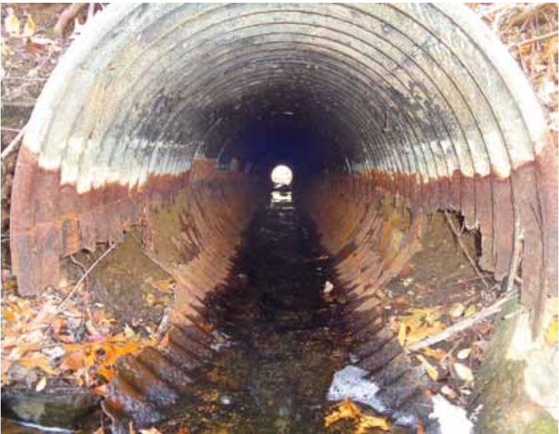
Photo 3. Example condition of a corrugated metal pipe culvert
