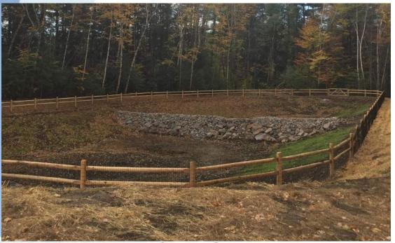
The Bartlett Brook Central Stormwater Treatment Wetland Shortly After Construction – The project included construction of the treatment wetland and drainage improvements to direct additional water to treatment. •Significant Reduction in Stormwater Flow To Bartlett Brook
