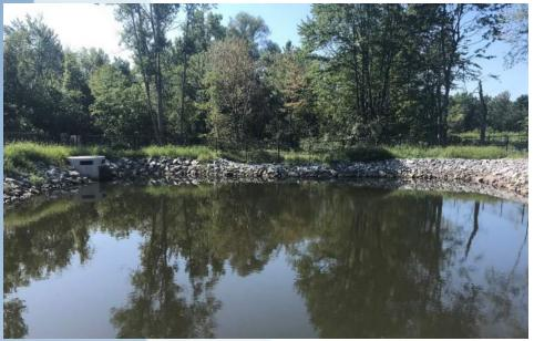
Commerce Square Detention Pond After Construction – The project included construction of the detention pond, installation of a swirl separator, and reconfiguration of drainage pipe to bring additional water to treatment.
