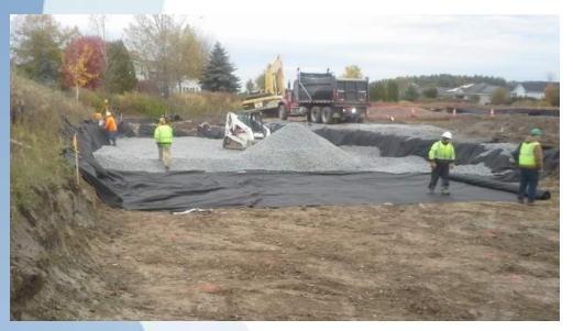
Placing Stone As Part of Treatment Wetland Construction – Project included retrofit of two existing stormwater ponds to stormwater treatment wetlands, and retrofit of two existing stormwater detention ponds to meet current standards
