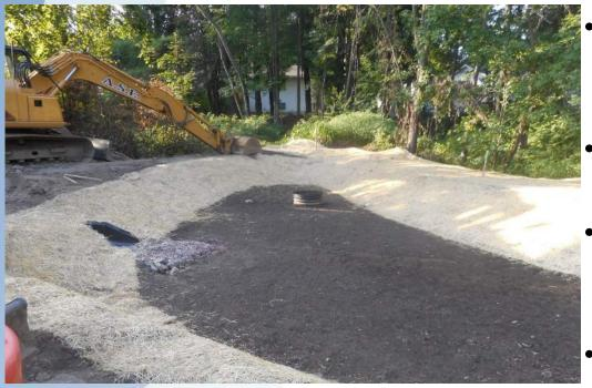
Iby Street Gravel Wetland During Construction – Project included construction of a small gravel wetland at the entrance to Dumont Park. Stormwater from the street and neighborhood previously discharged untreated to Potash Brook
