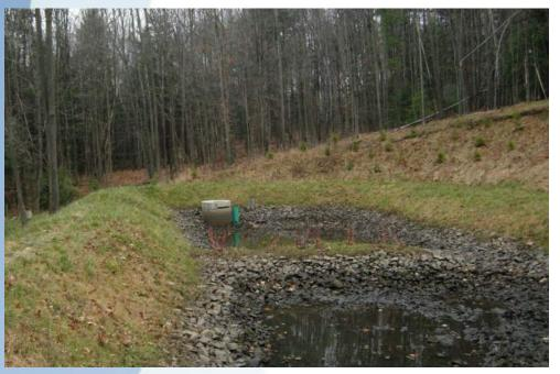
Existing Kennedy Drive Pond 3 – Retrofit and expansion of the Kennedy Drive Pond to a treatment wetland will provide better treatment of stormwater to a larger drainage area
