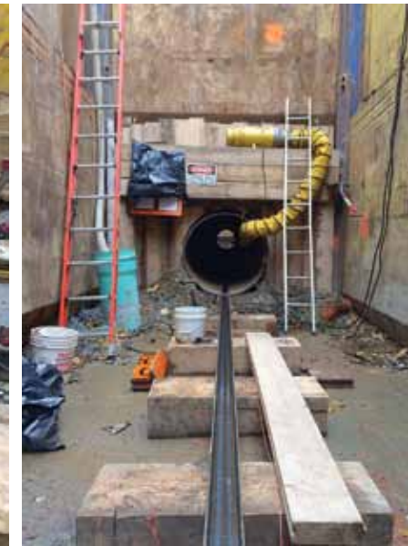
Installed 42 in. (1,067 mm) casing
