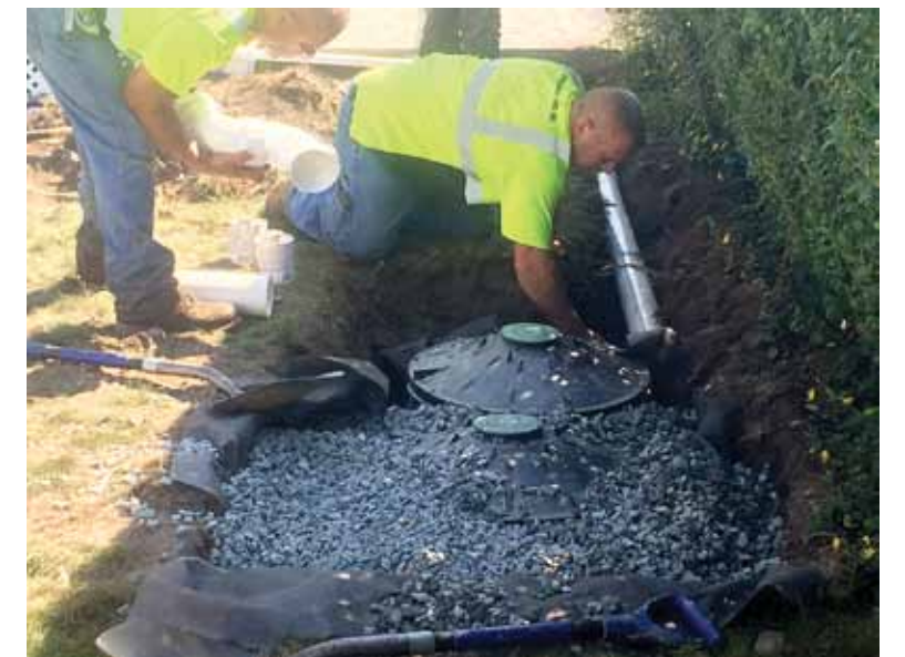
Installation of an infiltration basin
