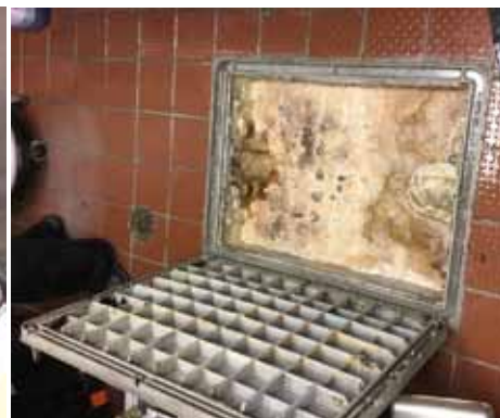
The second round of inspections found many FSEs in compliance with FOG requirements (left) and others violating the required cleaning frequency (right)
