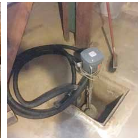
Sump pump that can be connected to the washing machine discharge piping
