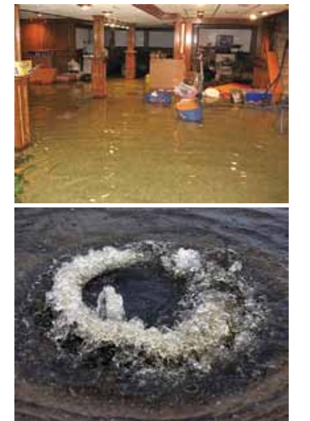
Impact of inflow—flooded basements and gushing manholes
