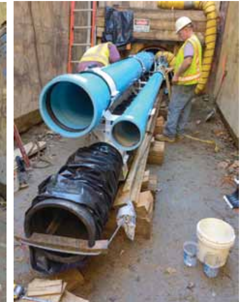
Casing spacers and triple pipe arrangement
