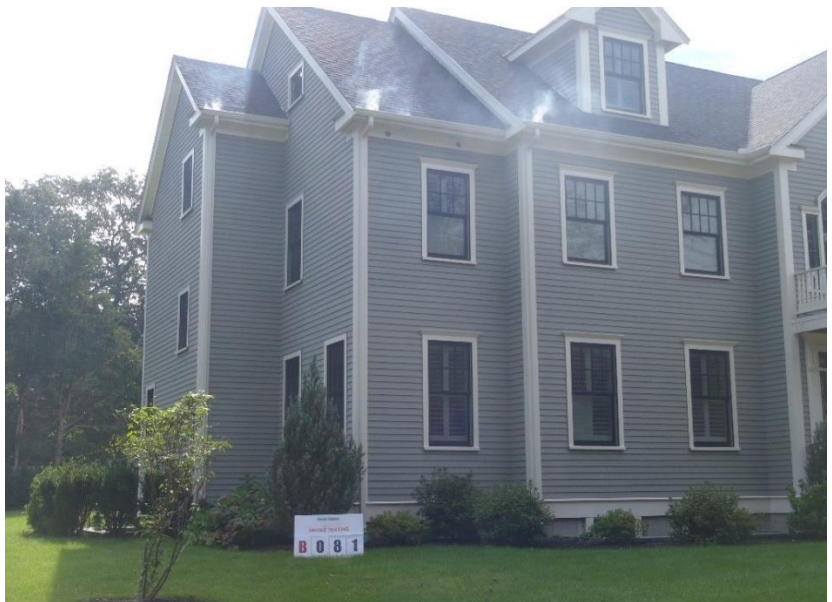
Photo 2 - Sample of Illicit Connection identified during Smoke Testing (Roof Leaders to Sewer - Image by Weston & Sampson)
