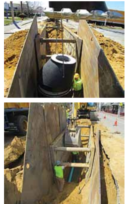
1. (top) Main Street sanitary manhole installation 2. Main Street gravity sewer installation
