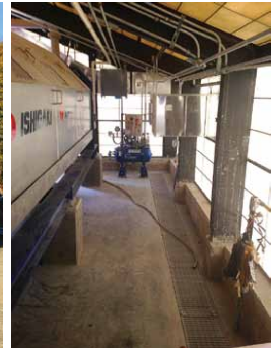
9. Trench drain running the length of the press
