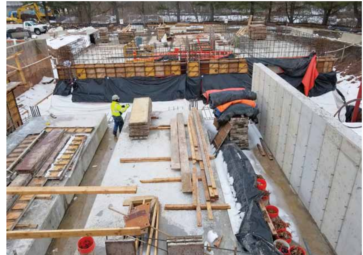
Plainville's new filter building in construction as of February 2019. Equipment pads for the disc filters are in the foreground. The background shows the flow equalization tank, which will be located underneath the chemical storage room.
