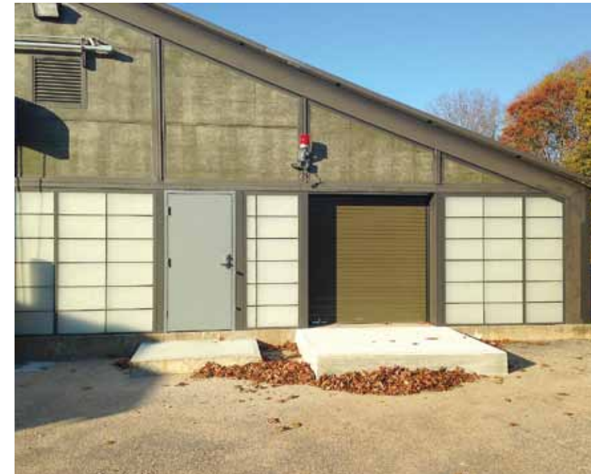
8. Platform outside the rollup door for polymer deliveries
