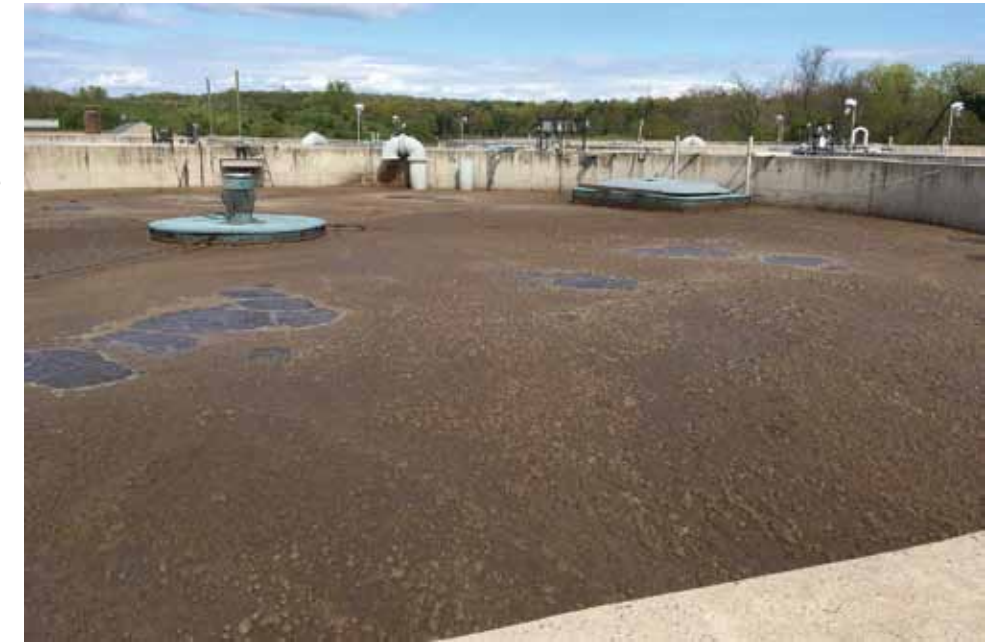
One of Plainville's SBRs in the react phase, showing the mixer on the left and the decanter on the right
