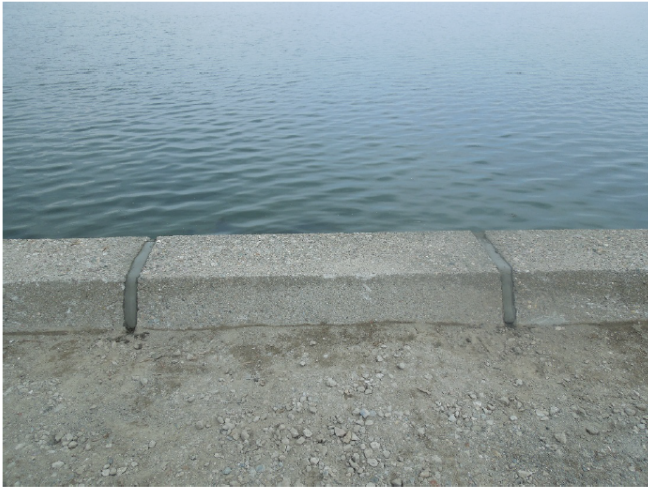
Roadside view of grouted joints along Dorchester Ave.
