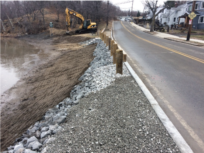
Revetment repair and curb reset at Nickerson Beach.
