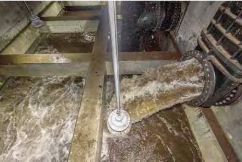
Field testing of rehabilitated pumps—view from interior of wet well
