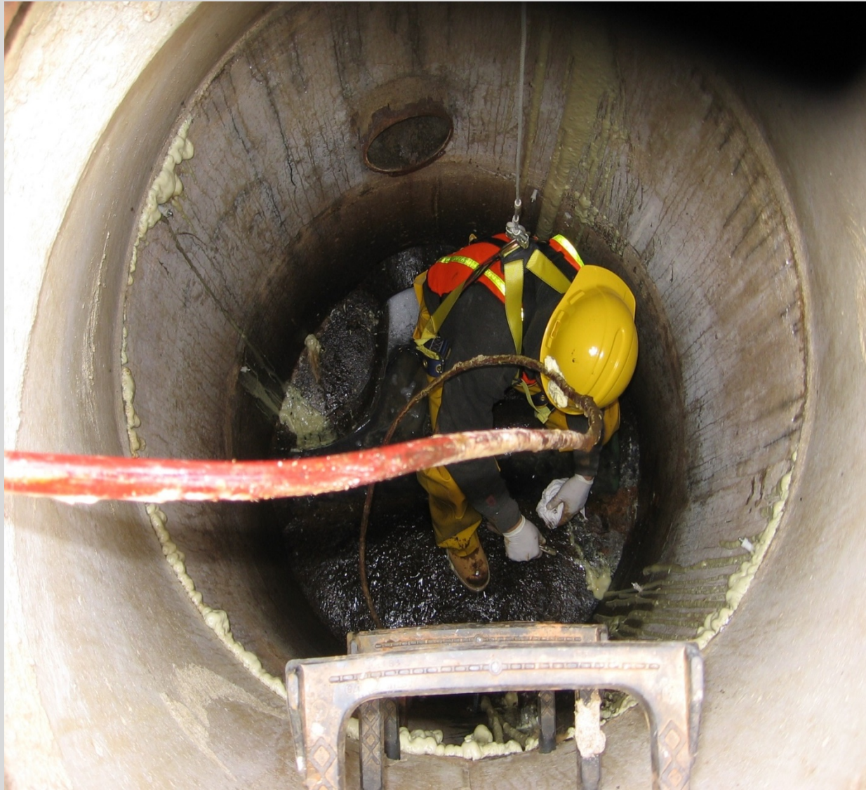
Sealing Pre Cast Manholes
