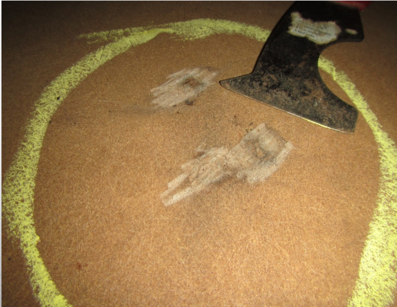
Staining in the eastern quadrant with scraped off gel coat - corrosion barrier intact
