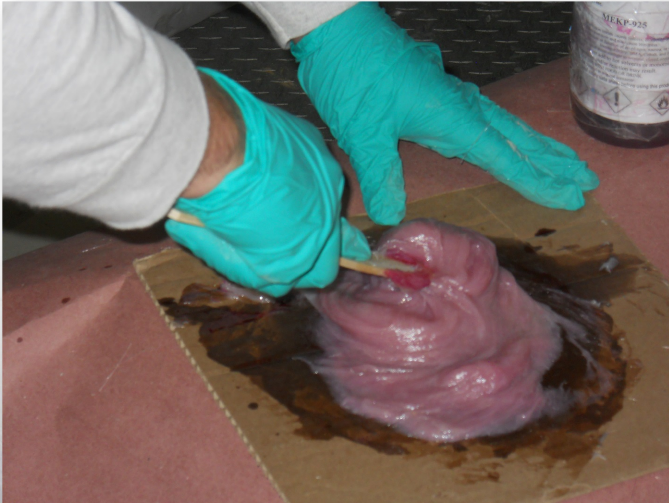
Depicts preparation of the vinyl ester resin repair compound
