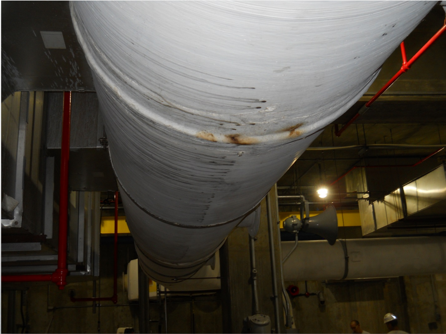
View of round ductwork on Grit Level – note leakage
