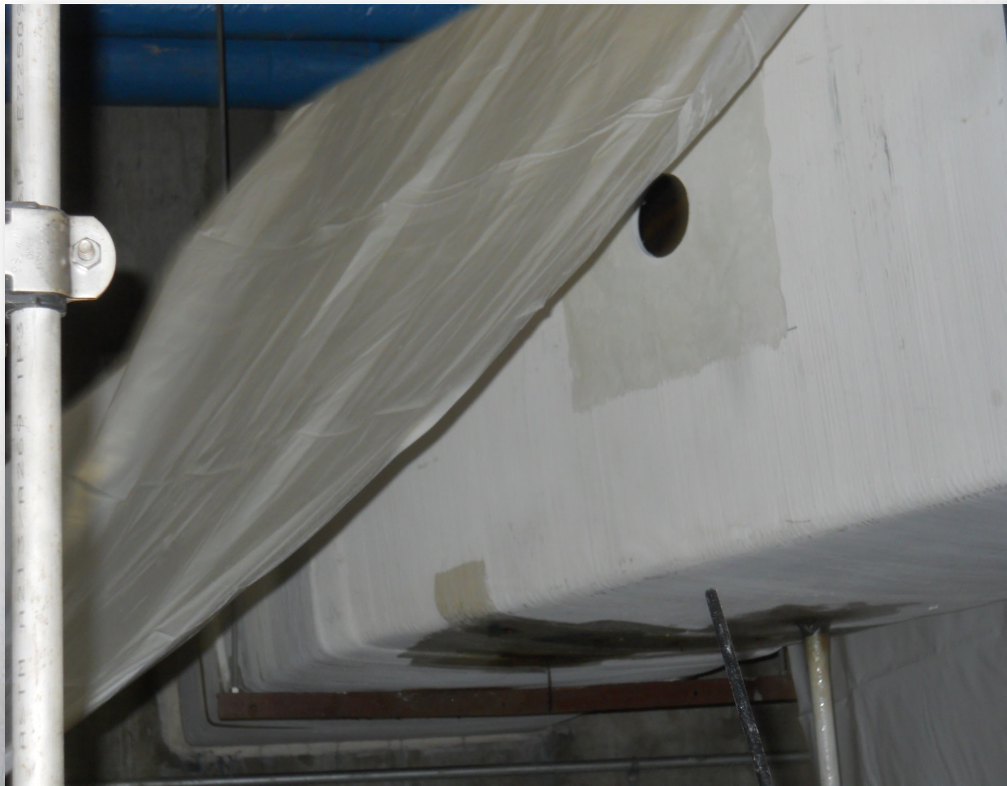
Shows the core hole in the duct – sample area
