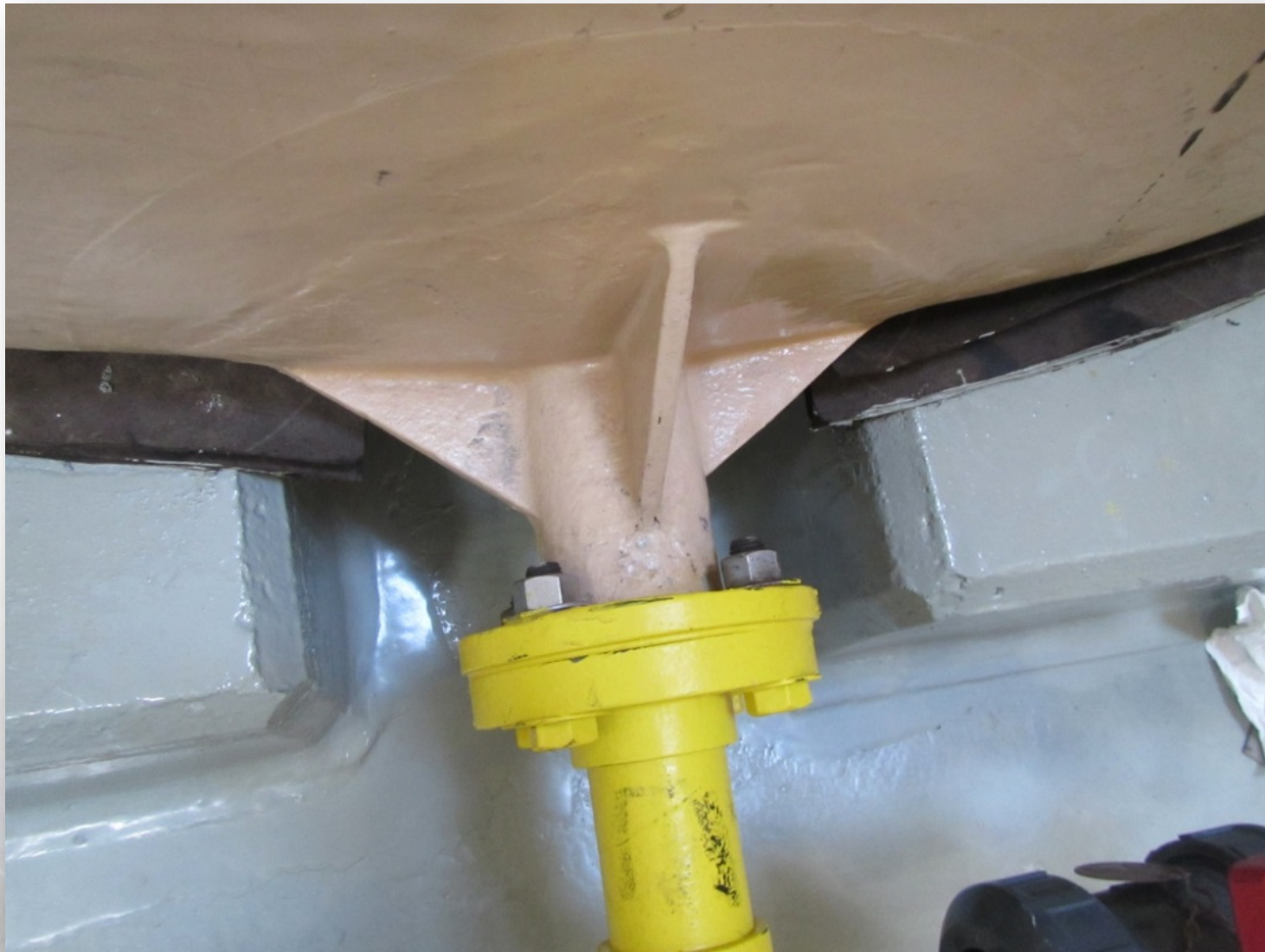
Gussets at tank drain pipe in the southwestern quadrant
