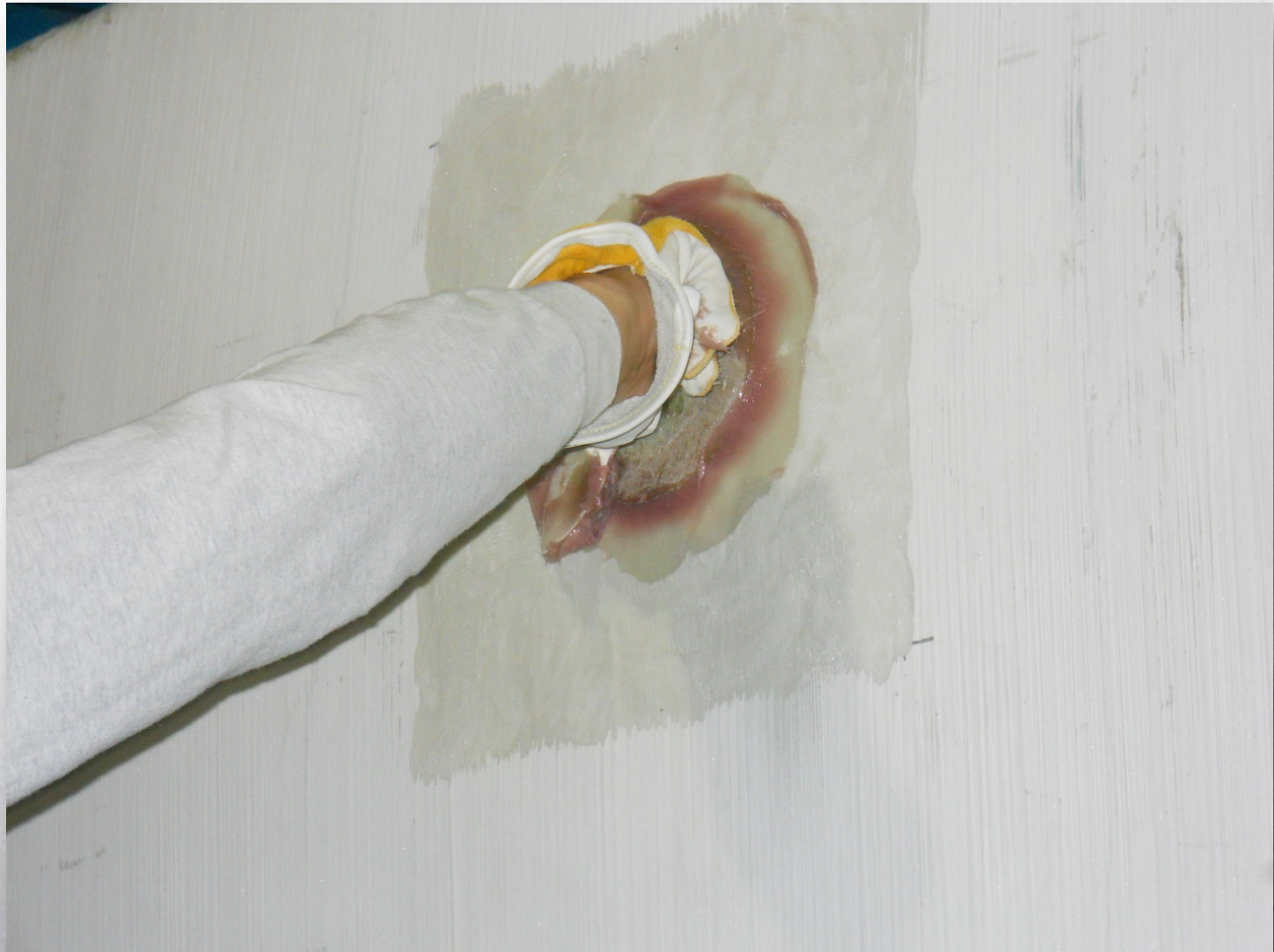
Demonstrates the flanged core hole repairs in progress
