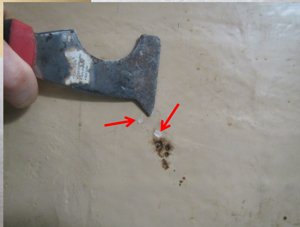
Detail of stain/burn marks in the northern quadrant of the tank interior
