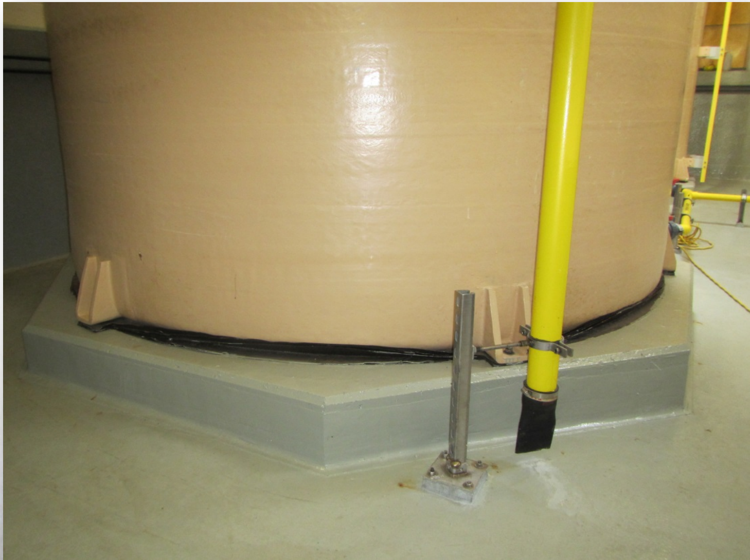
Concrete tank base, containment area and protective coatings
