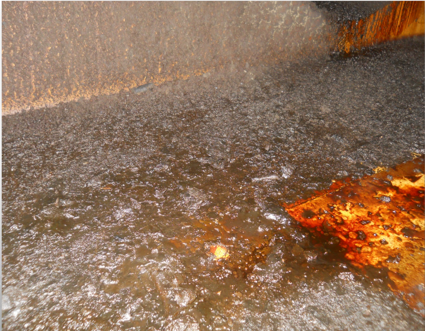
Abrasion damage to corrosion barrier
