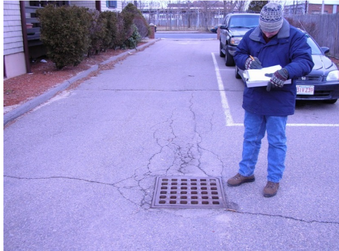
Parking Lot Drainage
