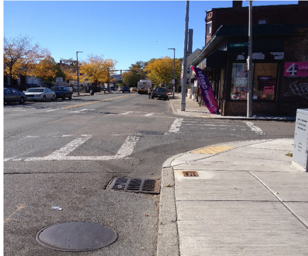
Roadway Catch Basins
