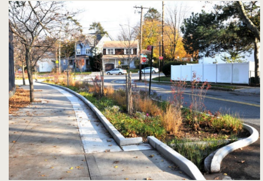
STORMWATER GREEN STREETS / BUMPOUTS
