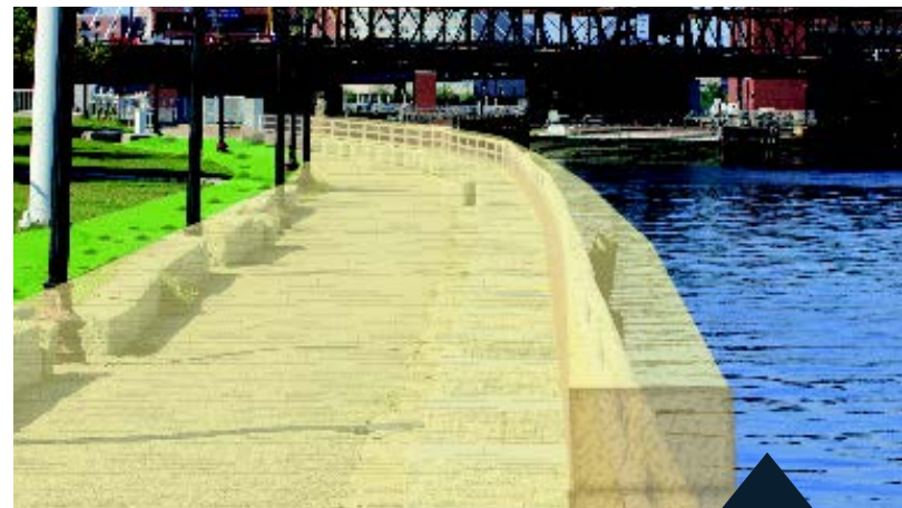
HARBORWALK FLOOD BARRIER
