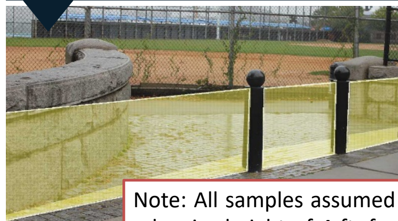
TEMPORARY FLOOD BARRIERS
