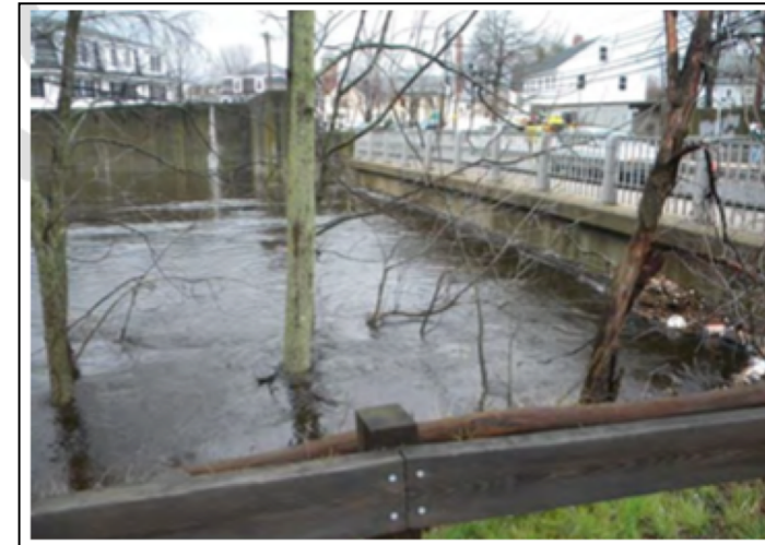
Sudbury River at Concord Street bridge during March 2010 storm
