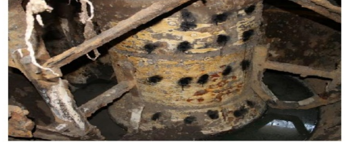
Photo No. 7 Center Column of Thickener No. 1, looking South at locations 1 and 16 thru 20.
