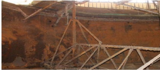
Photo No. 4 Wall of Thickener No. 1, under Skimmer Scum box, thin wall plate detected.
