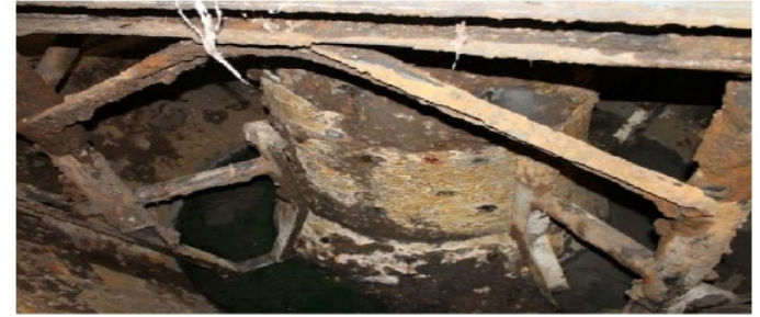
Photo No. 5 Center Column of Thickener No. 1, looking North at locations 10 thru 13.
