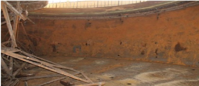
Photo No. 6 Wall and floor of Thickener No. 1, looking Southwest at locations 10 thru 14.
