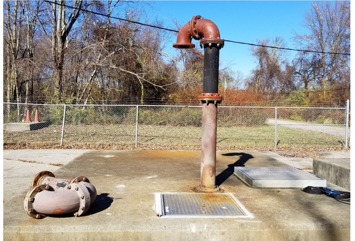
New Wet Well Access Hatch @ Knight St PS
