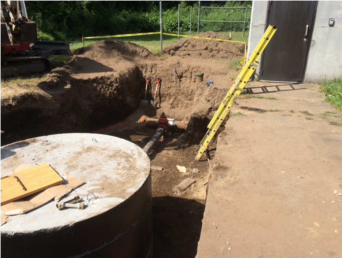
New Bypass Manhole & Force Main @ Knight St PS
