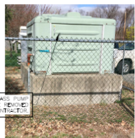
EX. FIBERGLASS PUMP SKID ENCLOSURE SCALE: NTS
