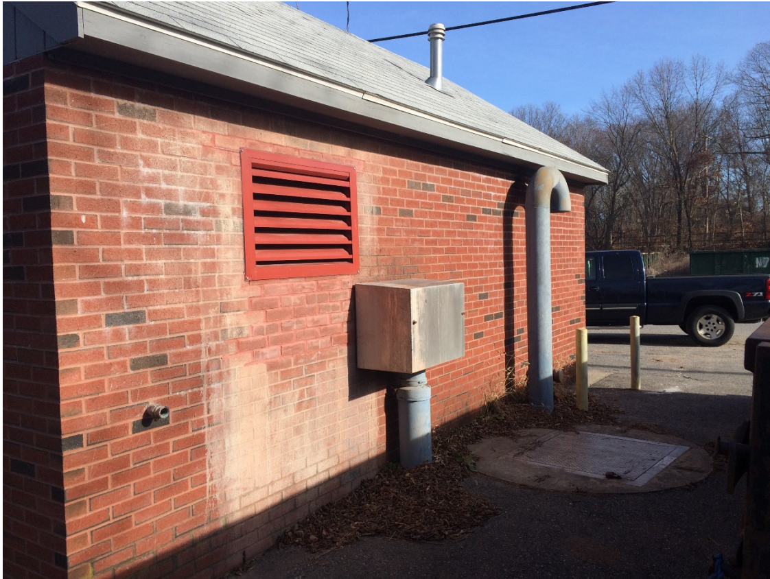
Exterior View of Relocated Intake Louver (East Natick I PS)
