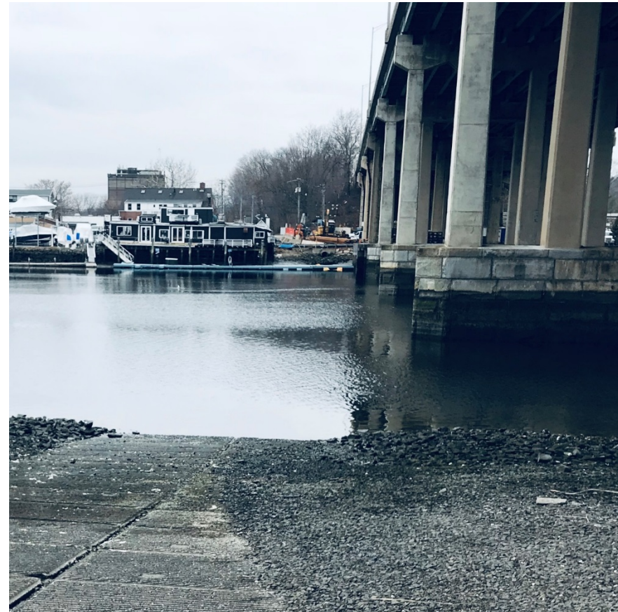
Looking east to west along the HDD alignment
