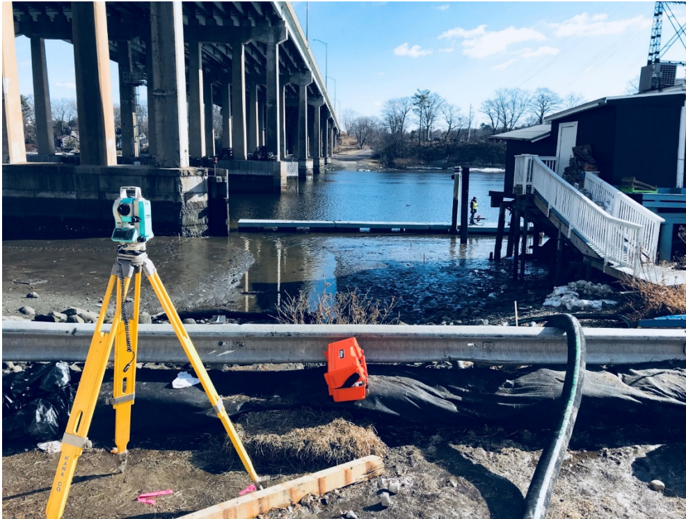
Looking west to east along the HDD alignment
