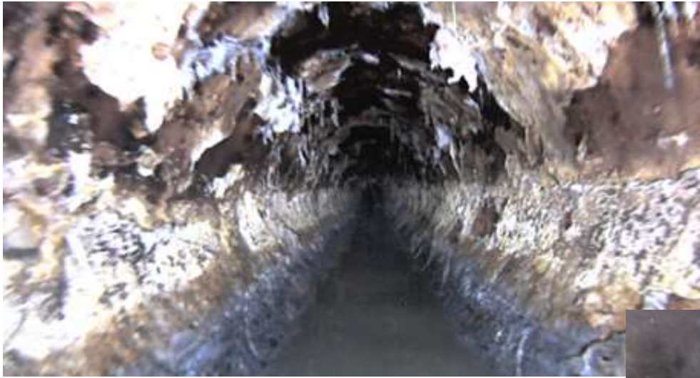
Liner delamination
