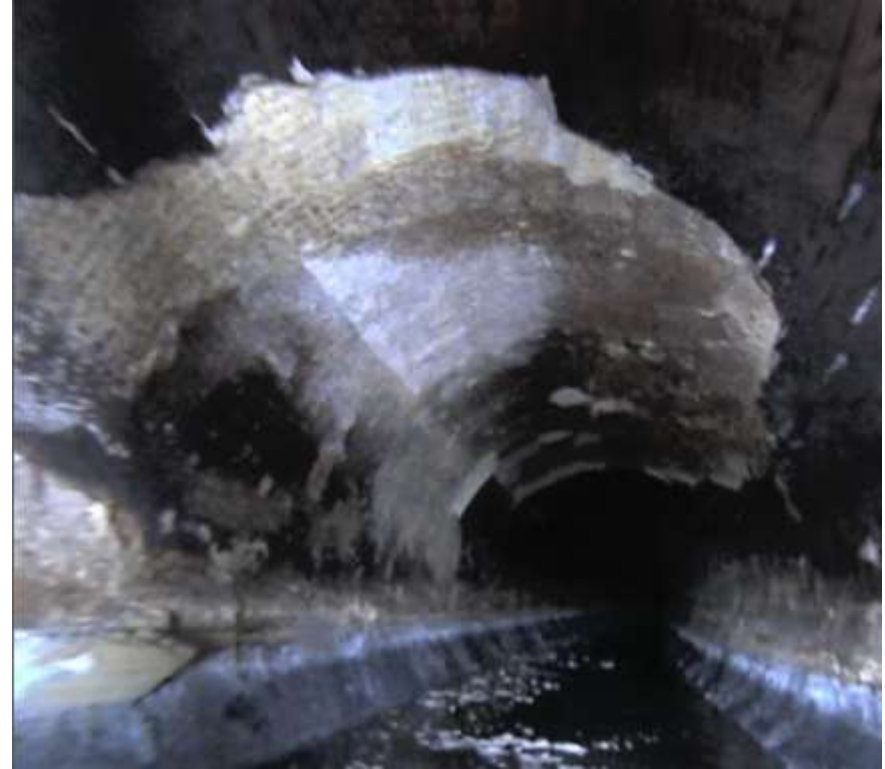
~25 LF of exposed rebar
