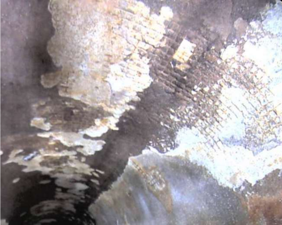
~35 LF of exposed rebar
