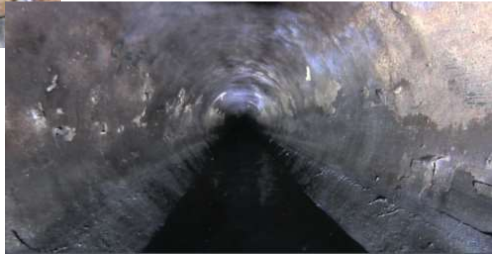
Surface spalling
