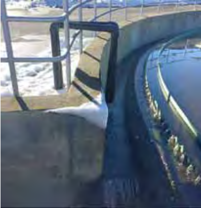
Photo 3. Dosing location into settling tank launder
