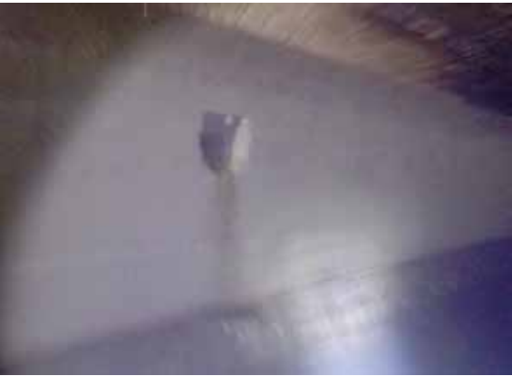
Photo 2. Lateral detected through drone inspections
