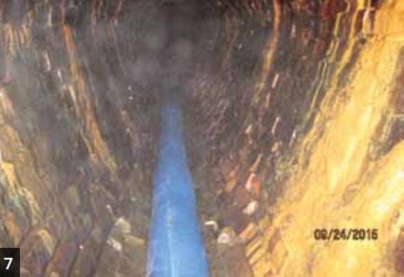
Photo 6. Cleaned and fully operational northern siphon barrel
