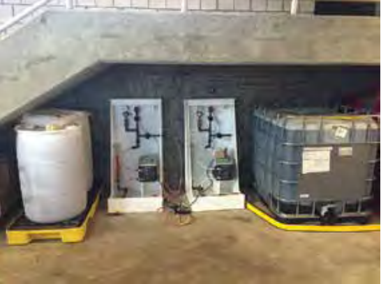
Photo 1. Temporary chemical feed pump skids and storage
