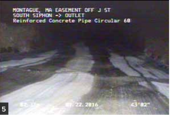
Photo 4. Deterioration of force main encasement in the siphon northern barrel
