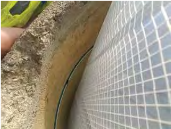
Photo 9. Installation of hydrophilic end seals and pre-liner and making its way into the manhole structures. The pre-liner was installed to help prevent resin washout in the CIPP liner during inversion and curing. Photo 9 depicts the end seals and pre-liner.
