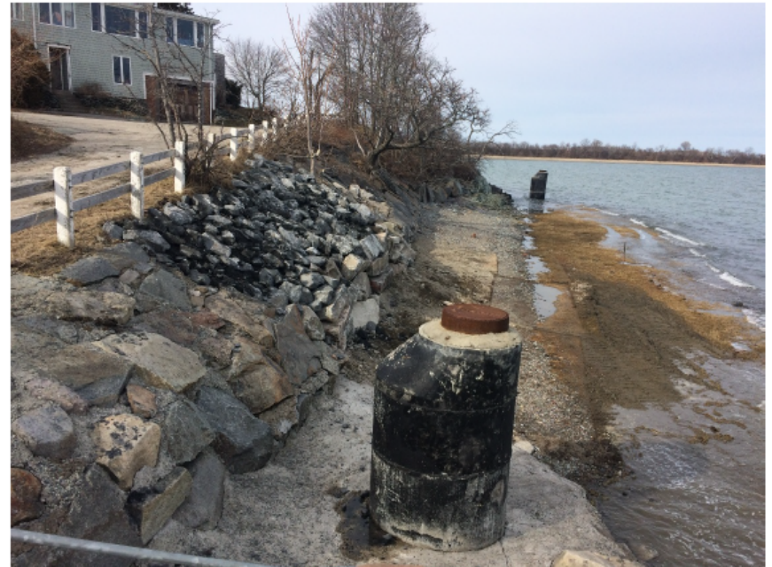
Revetment repair along Bayside Road.
