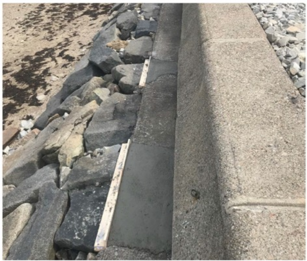
Leveling slab repaired at seawall along Shelton Rd.
