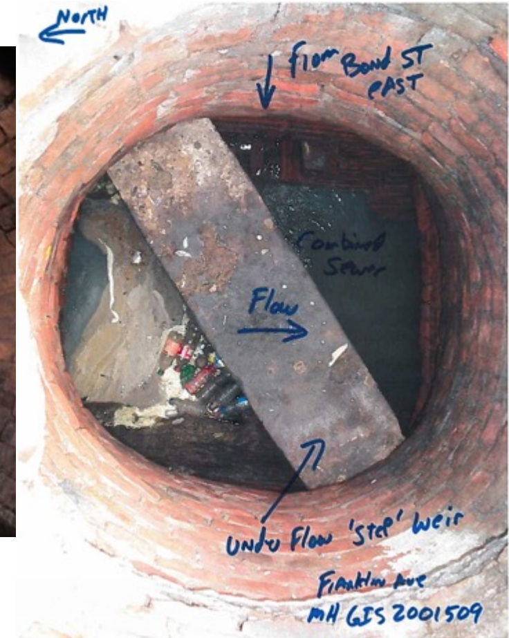
View from manhole
