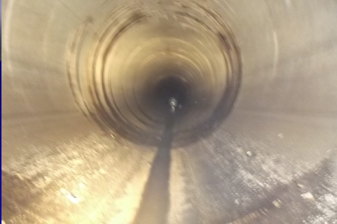
Tunnel – Looking Towards FP
