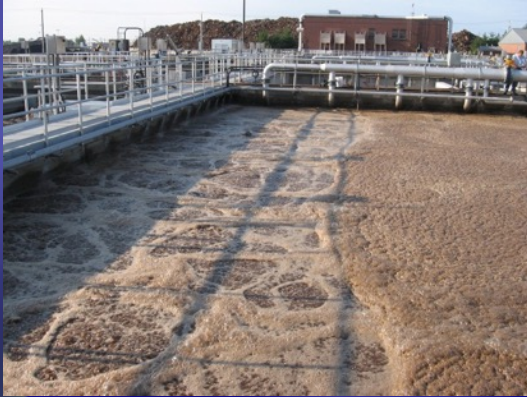
FP BNR Project 1,751 pieces of equipment
